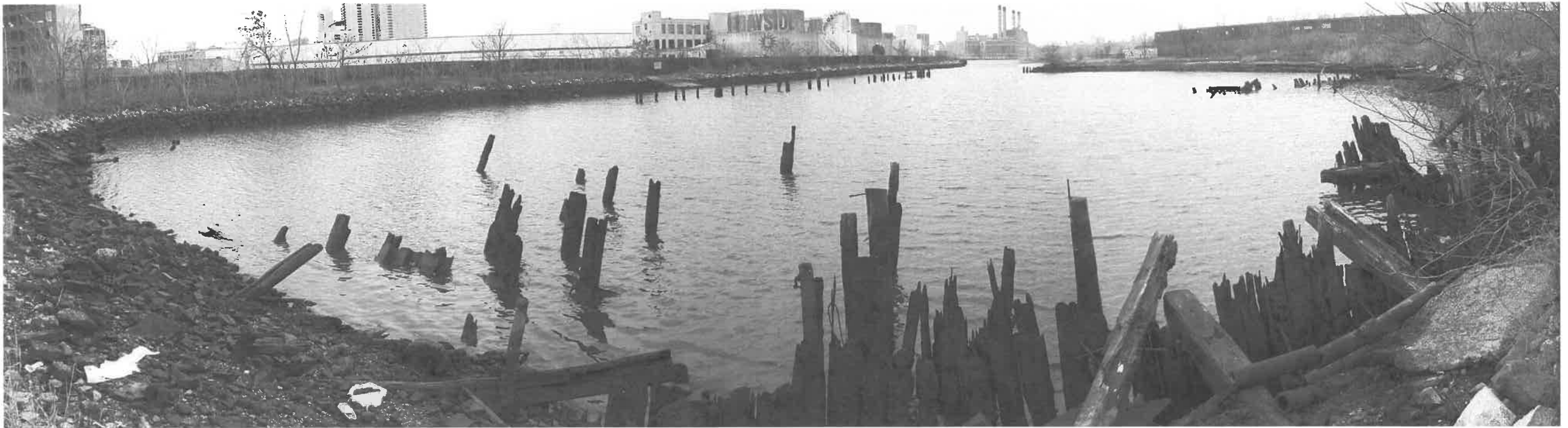
1 - Panoramic View of Existing Conditions
