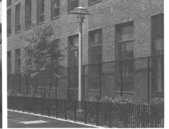
SECURITY LIGHTING- FLUSHING MEADOWS LUMINAIRE & POLE [GREENPOINT-WILLIAMSBURG MASTERPLAN STD., 12'-0" HT. 'B-POLE' AND 'RIVERSIDE PARK LUMINAIRE' COLOR: SILVER
