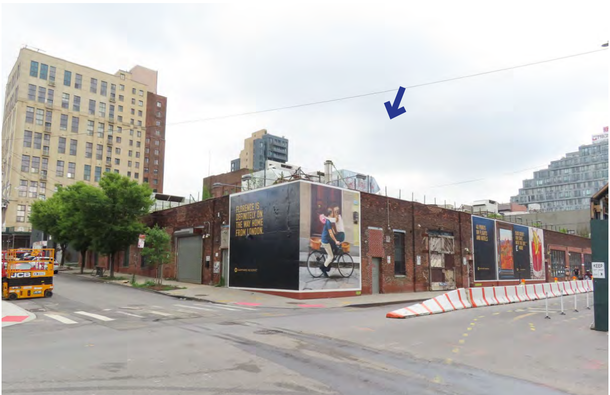
C. View of Development Site facing southeast from the intersection of Kent Avenue and South 1st Street.
