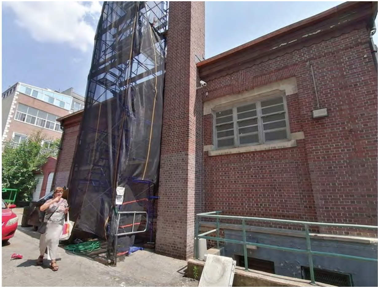
PHOTO 7: EXISTING VIEW OF EAST ELEVATION
