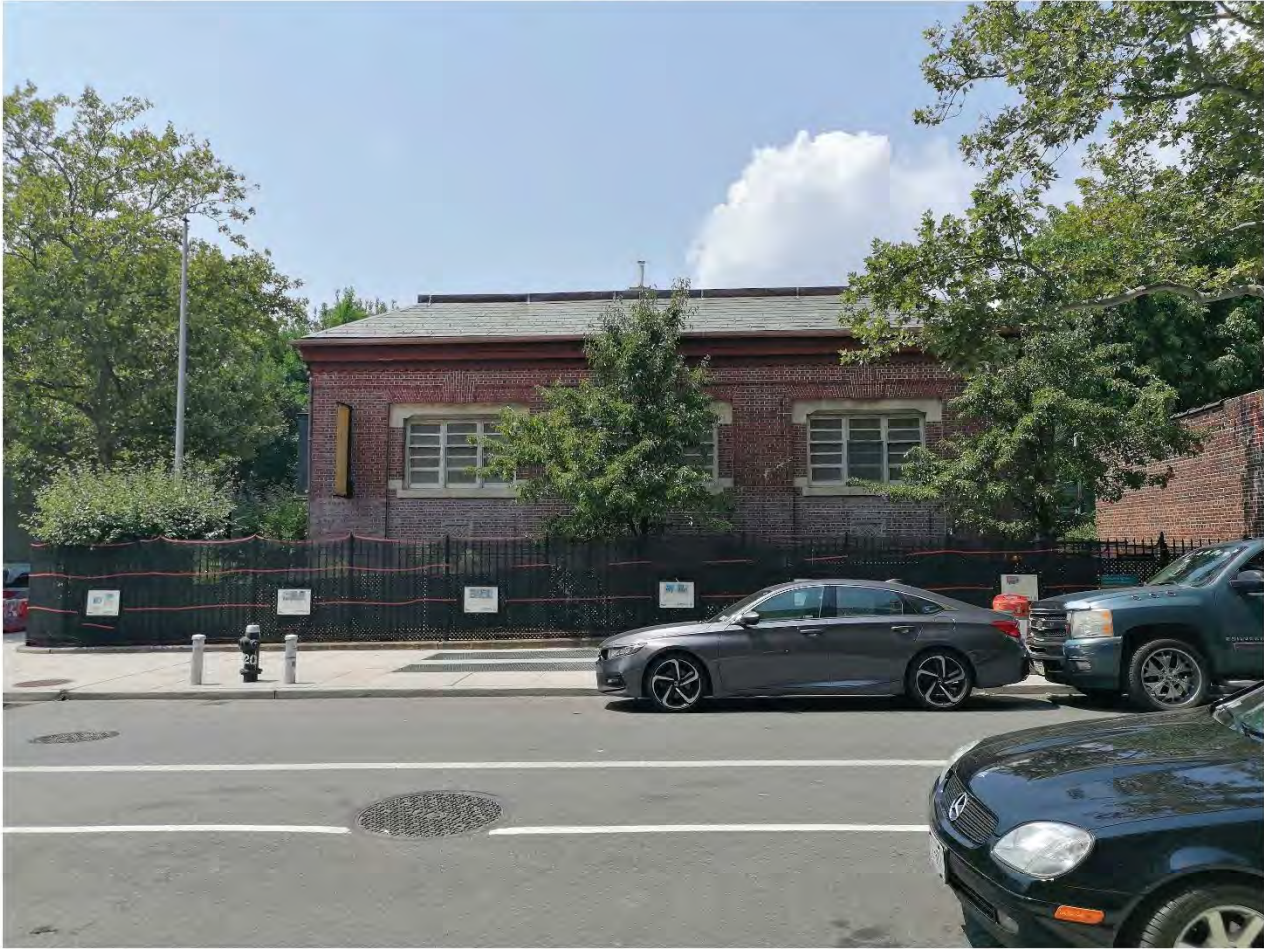
PHOTO 4: EXISTING VIEW AT EAST FACADE AT LEONARD STREET
