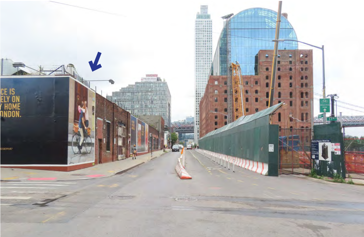
A. View of Kent Avenue facing Southwest from South 1st Street. (Development Site at left)
