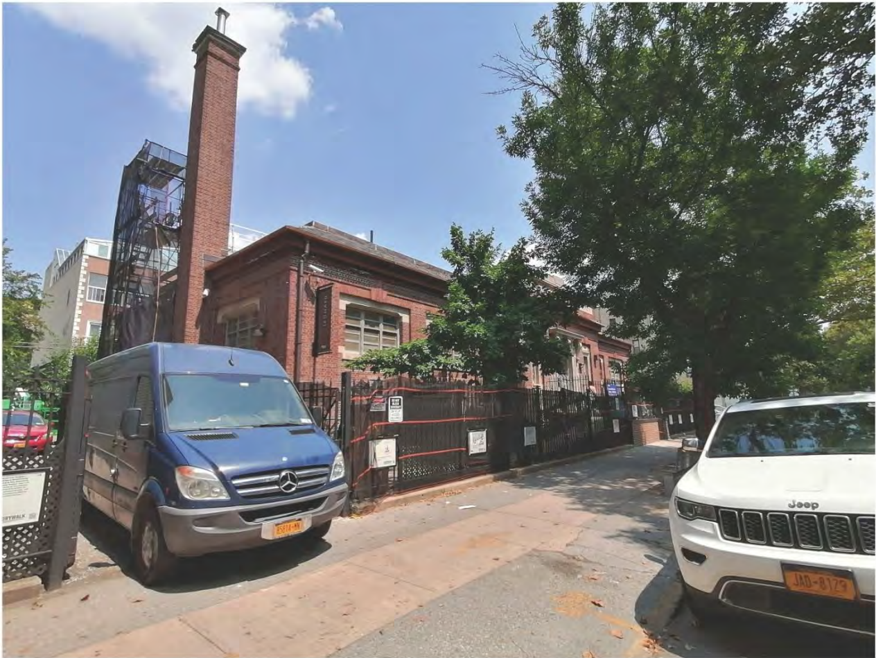
PHOTO 2: EXISTING VIEW OF ENTRANCE AT PARKING AREA
