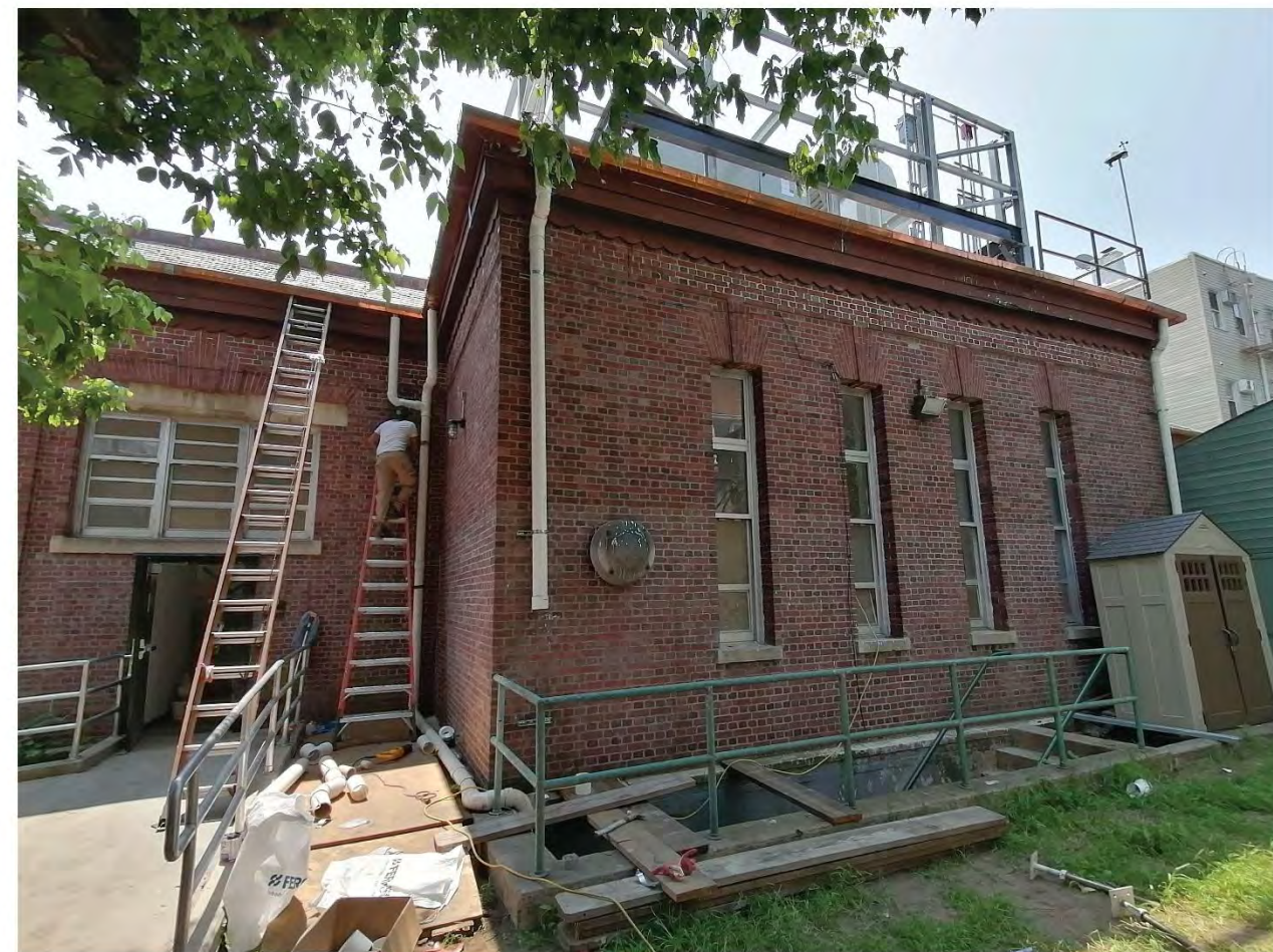
PHOTO 6: EXISTING VIEW OF REAR / NORTH ELEVATION
