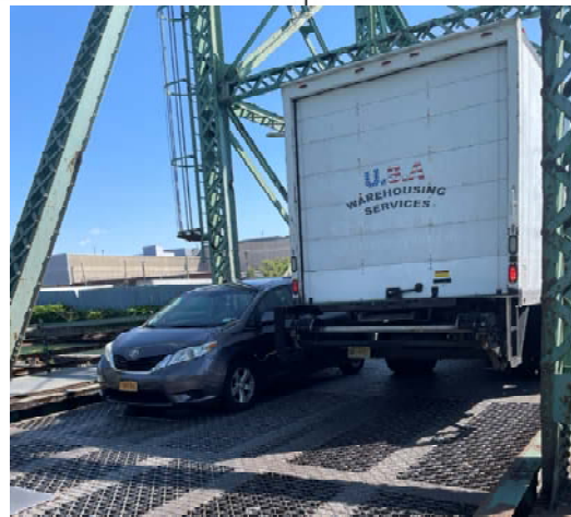
Typical Condition with Traffic on the Bridge
