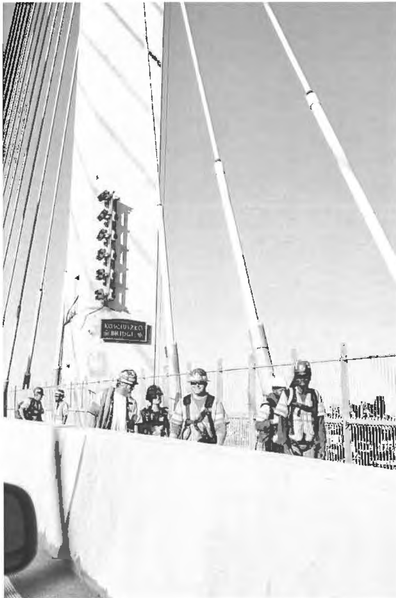
The new Kosciuszko Bridge is New York City's first cable-stayed bridge. Steel cables are placed at an angle to connect the bridge deck to vertical towers. Gabby Jones for The New York Times
