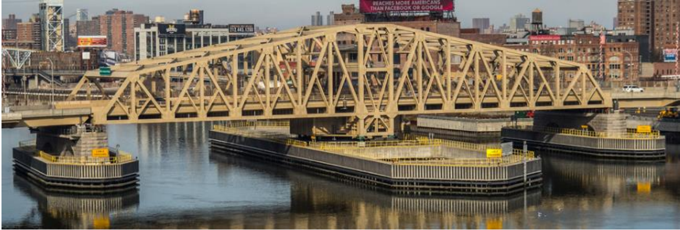
Willis Avenue Bridge, NYC (Symmetrical Swing)
