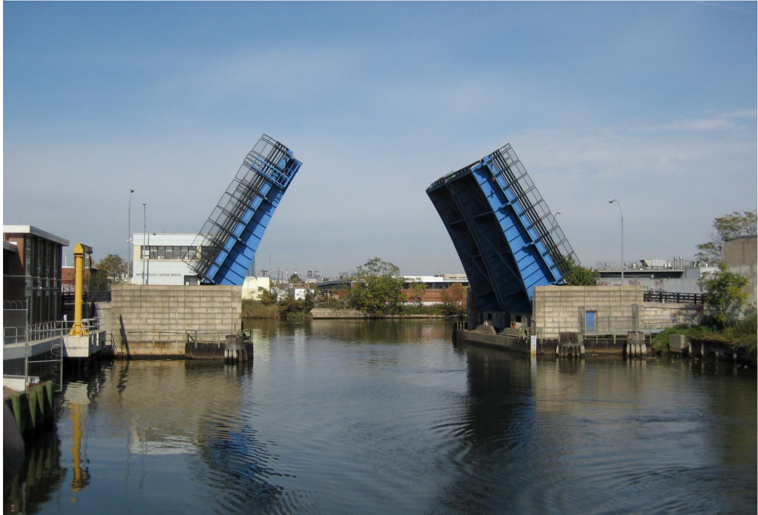
Metropolitan Avenue Bridge, NYC
