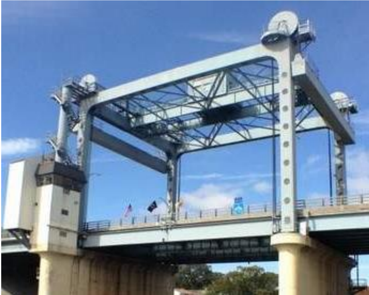
Lovelandtown Bridge, NJ
