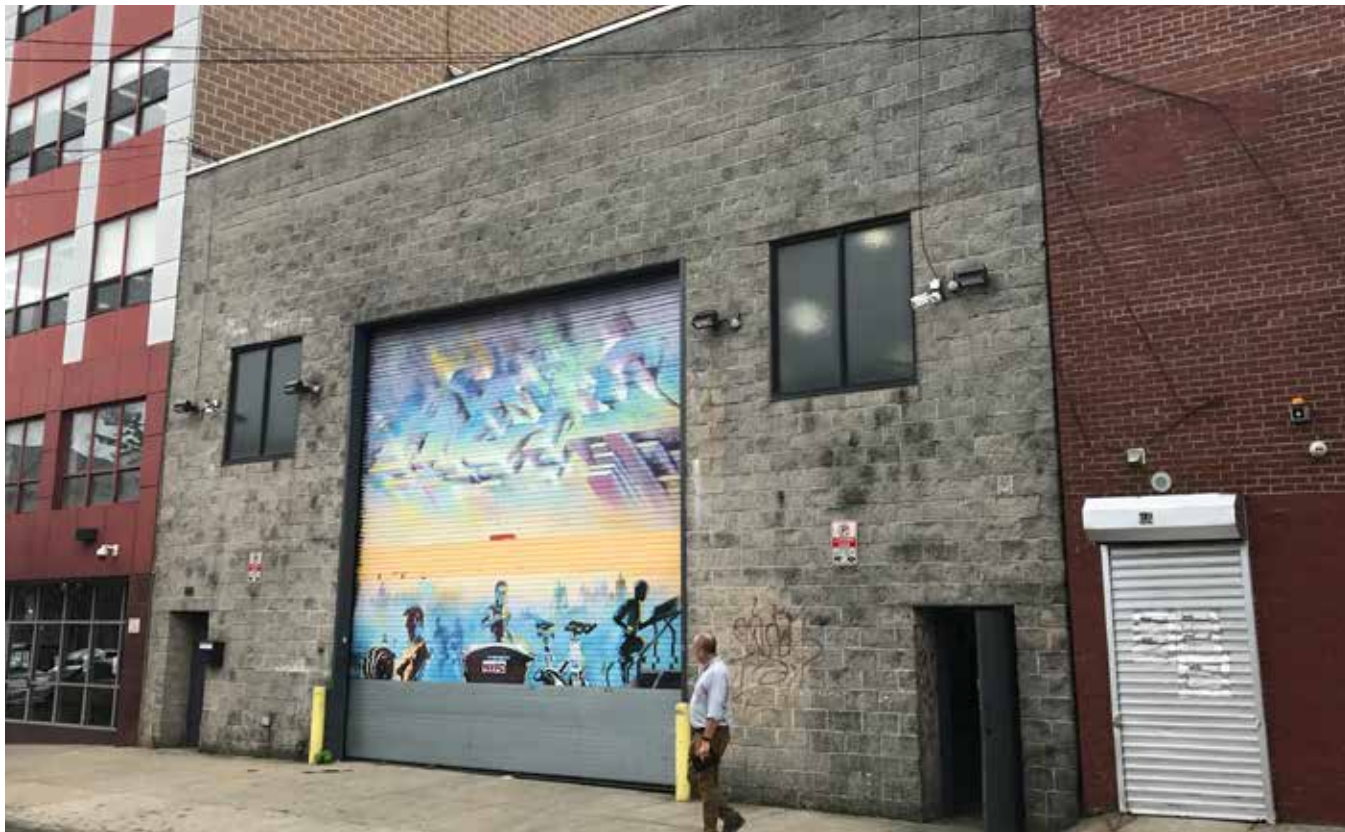
North/ Front Facade
