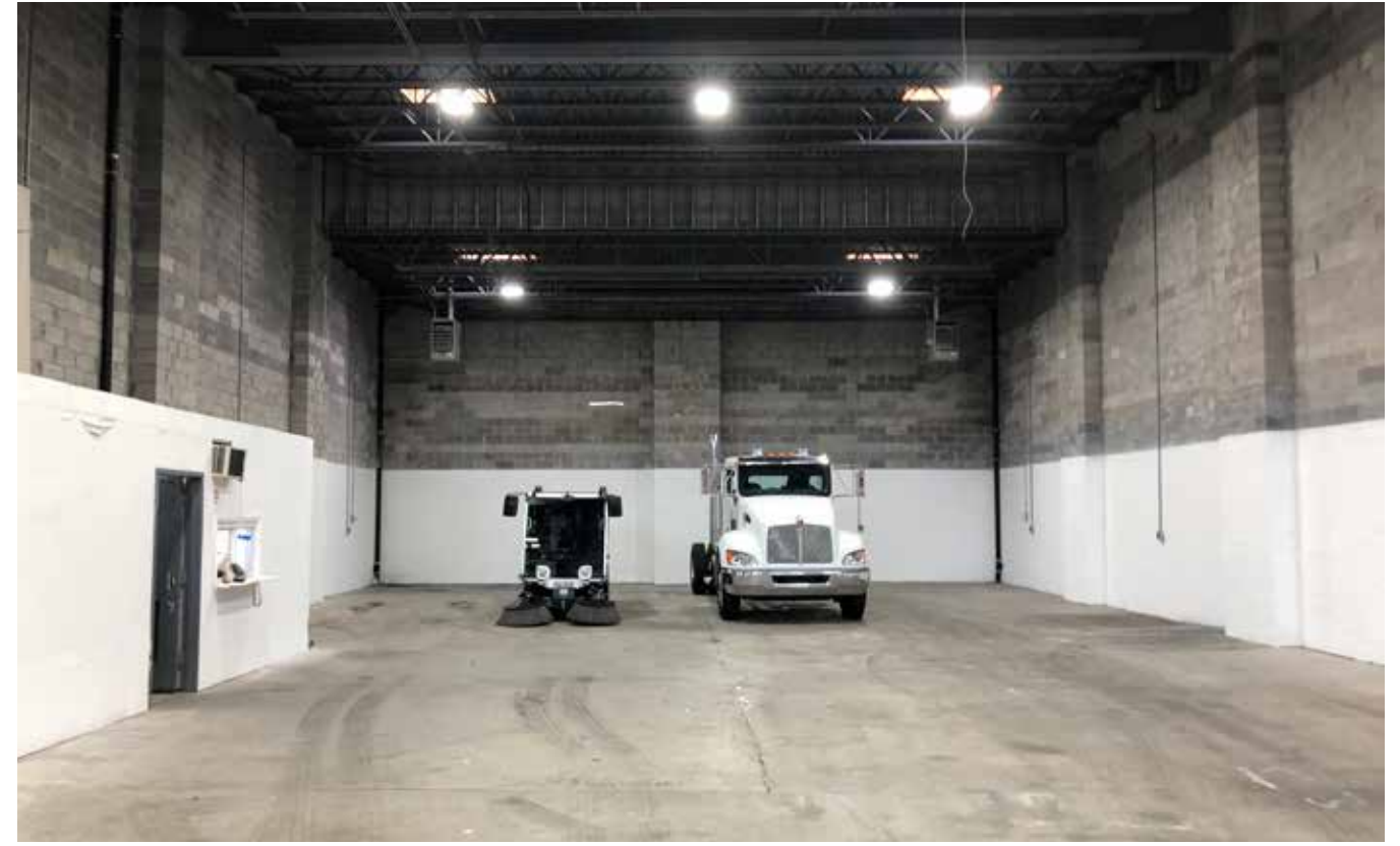
Interior View looking South
