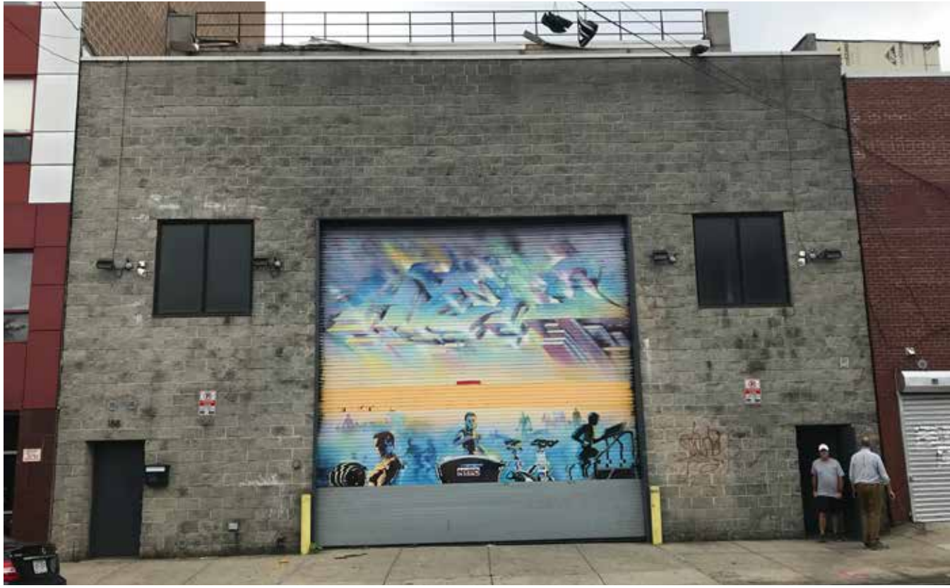
North/ Front Facade
