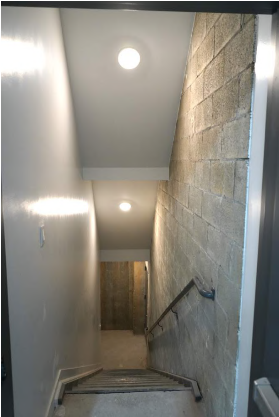
Image looking down the stairs into the cellar from ground level
