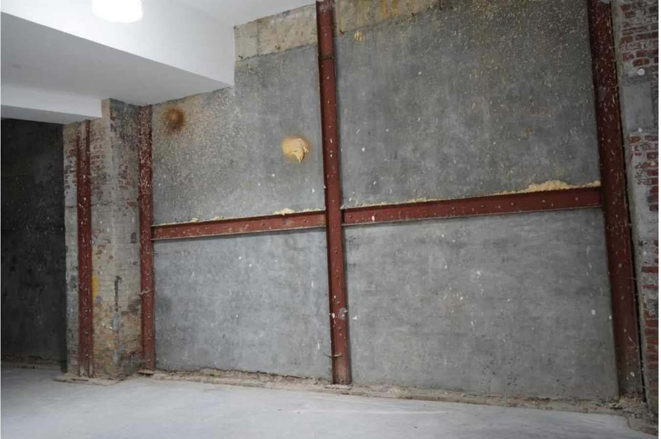
Image of bar location farther into the room, extending from the kitchen facing South/West
