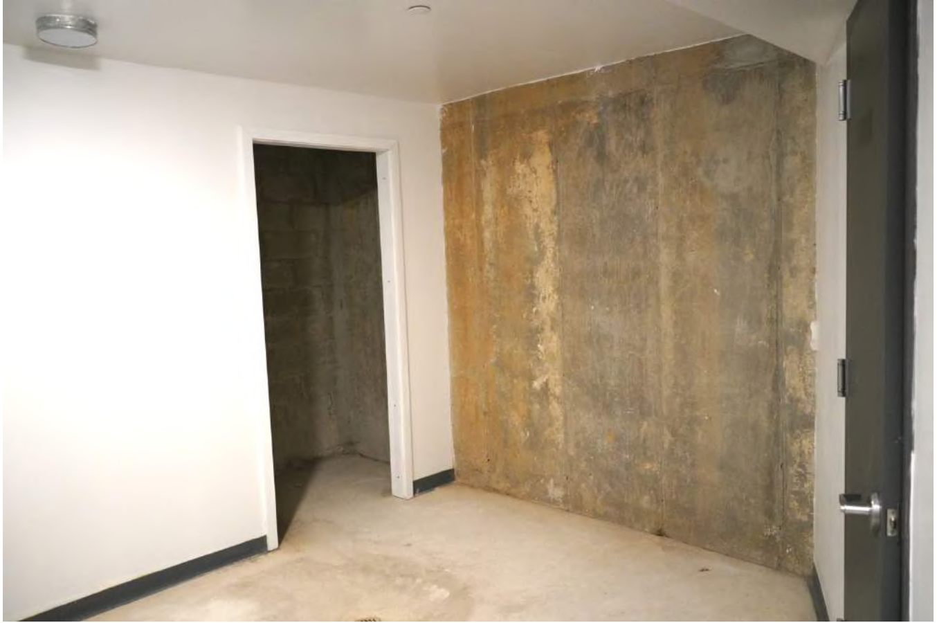
Image of storage room facing South
