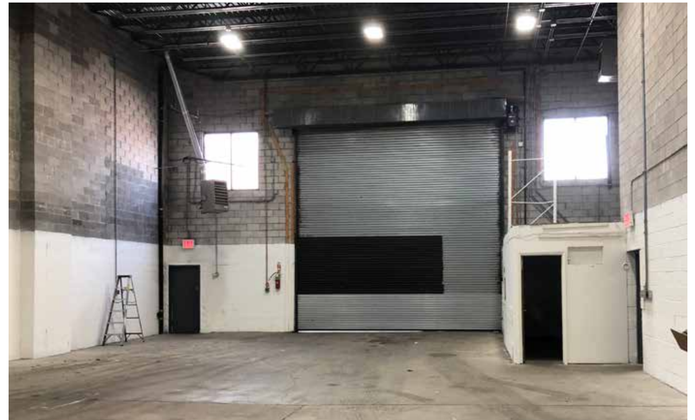
Interior View looking North
