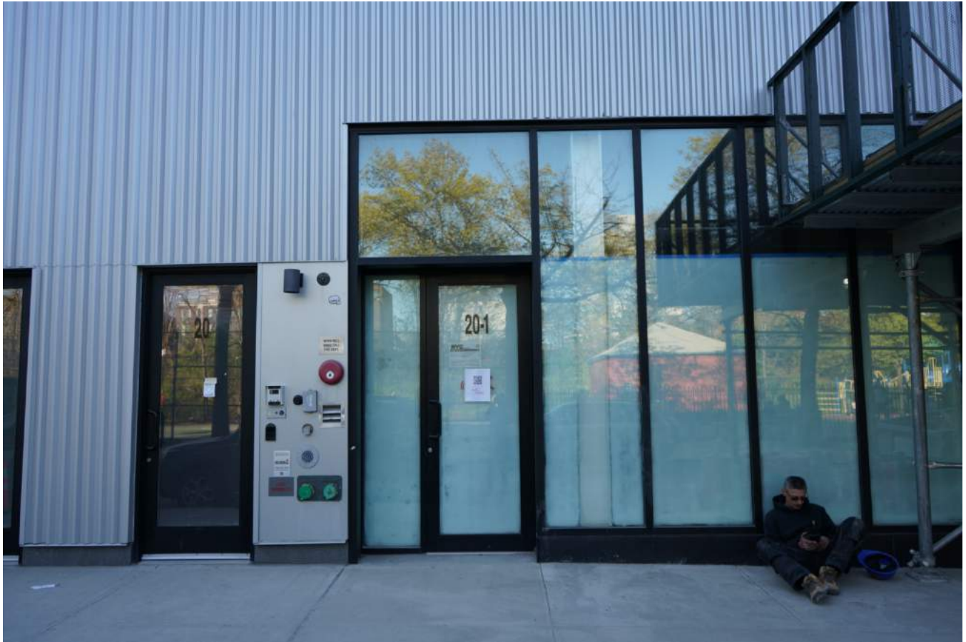
Front-facing image of café/bar at 20-1 with sidewalk facing West
