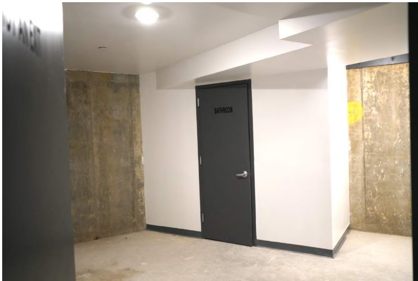
Inside hospitality storage room facing South/West
