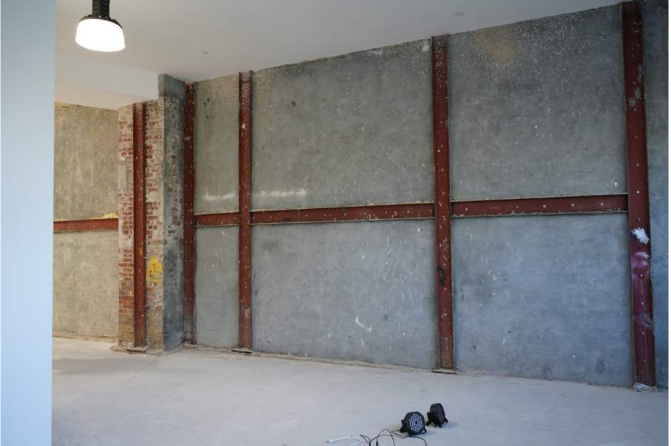
Image from entry facing the future electric kitchen area facing South/West
