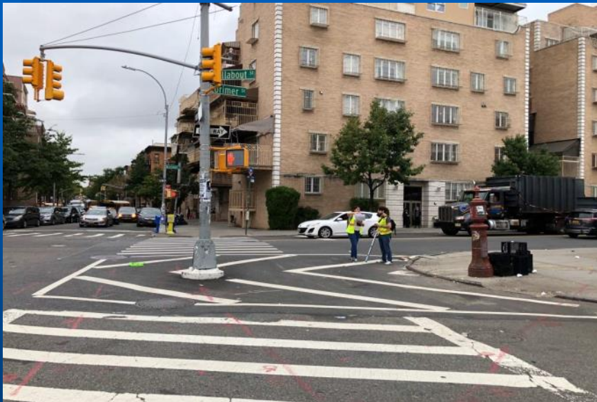
Existing channelized area- Concrete island to be built
