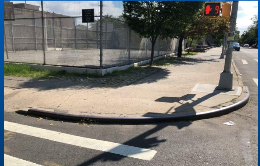
Existing corner to be reconstructed with new ramps
