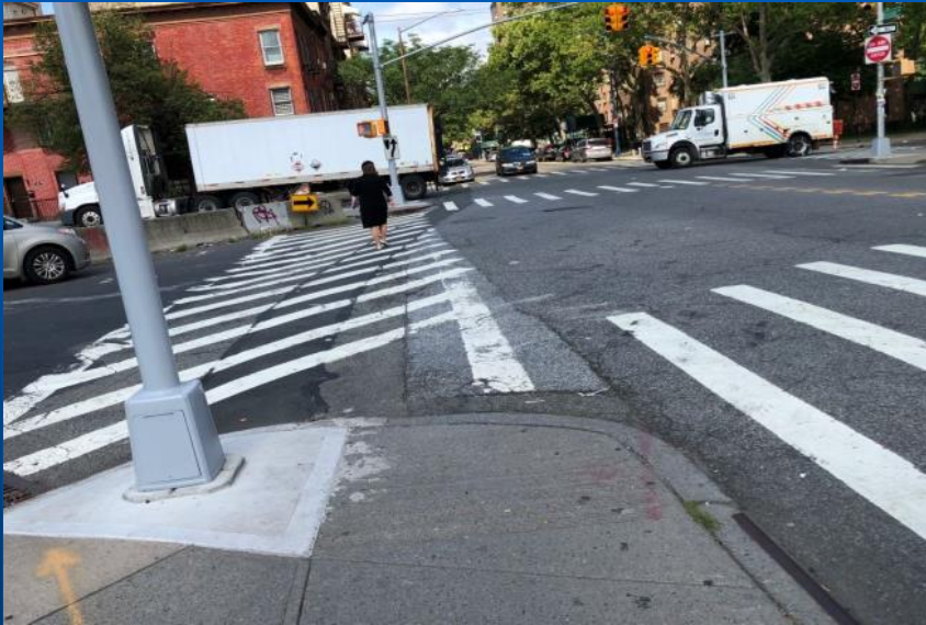
Existing corner to be reconstructed with curb extension and new ramps
