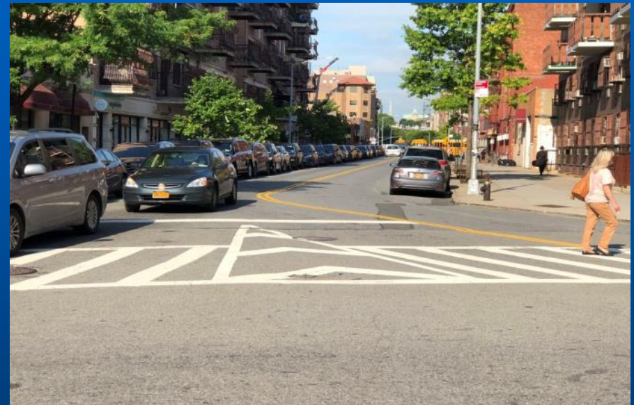
Existing channelized area- Concrete island to be built
