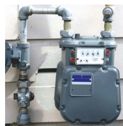
Gas meter with regulator and vent
