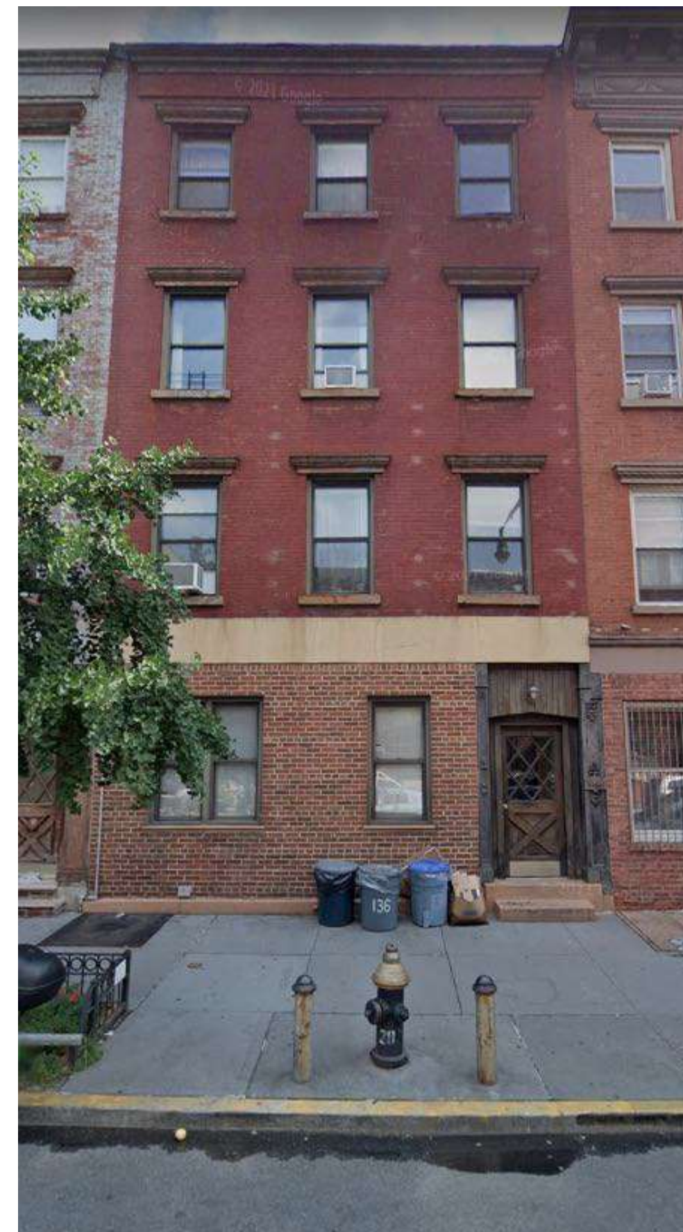
136 Franklin Street ( Existing Condition)
