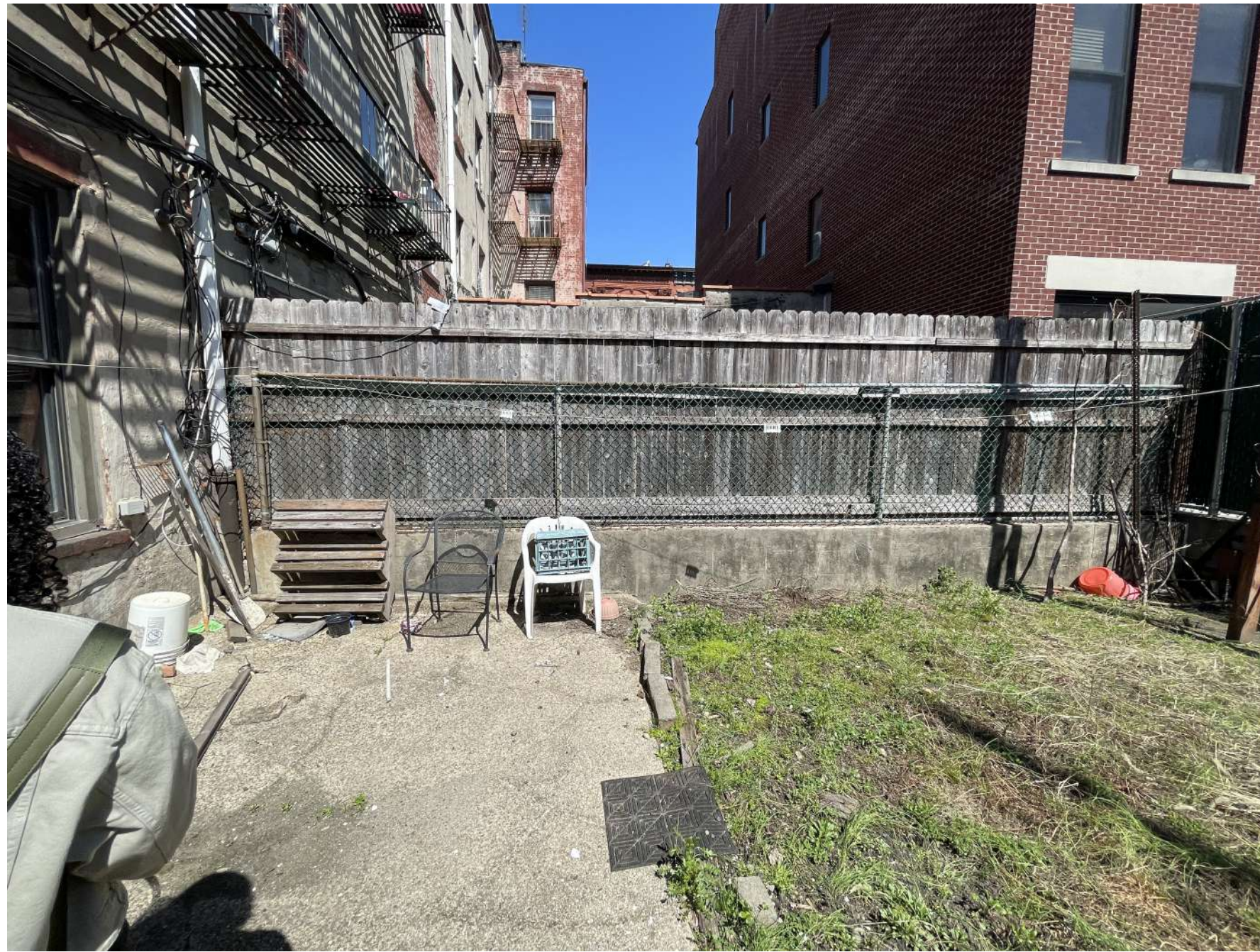
1 Current Rear Yard (View A) T-009.00
