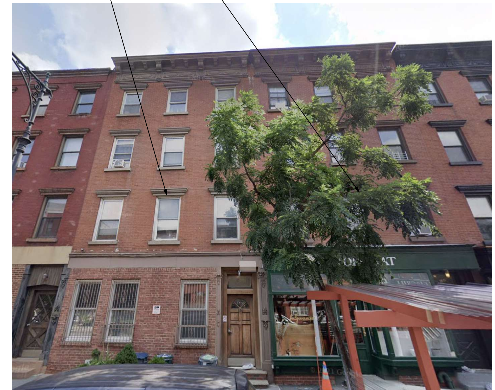
Existing Building w/ Balconies (View At Franklin Street)
