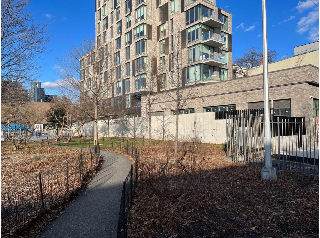
Concrete wall (160'w x 8'h) spanning the eastern border of the park.
