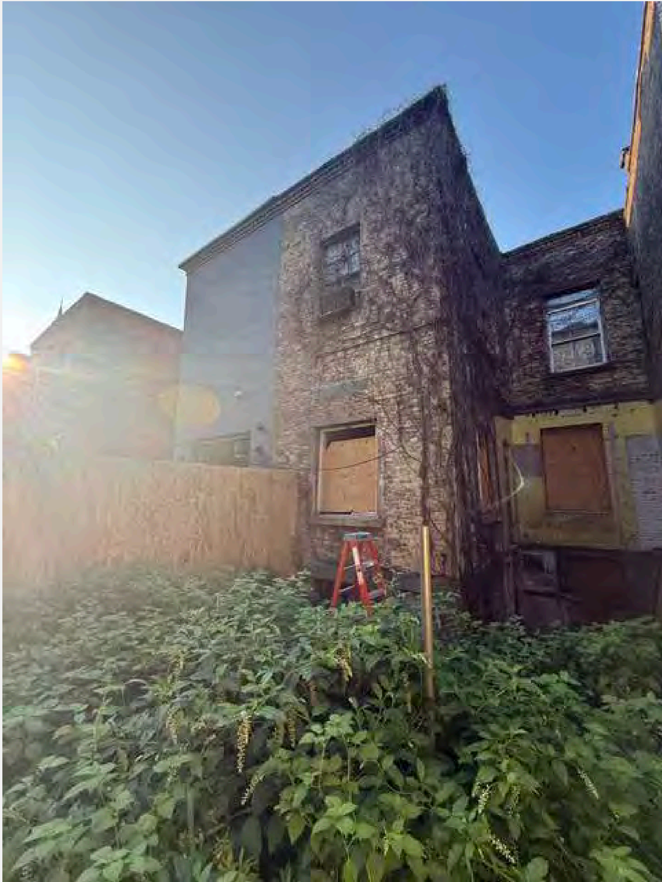
EXISTING REAR FACADE
