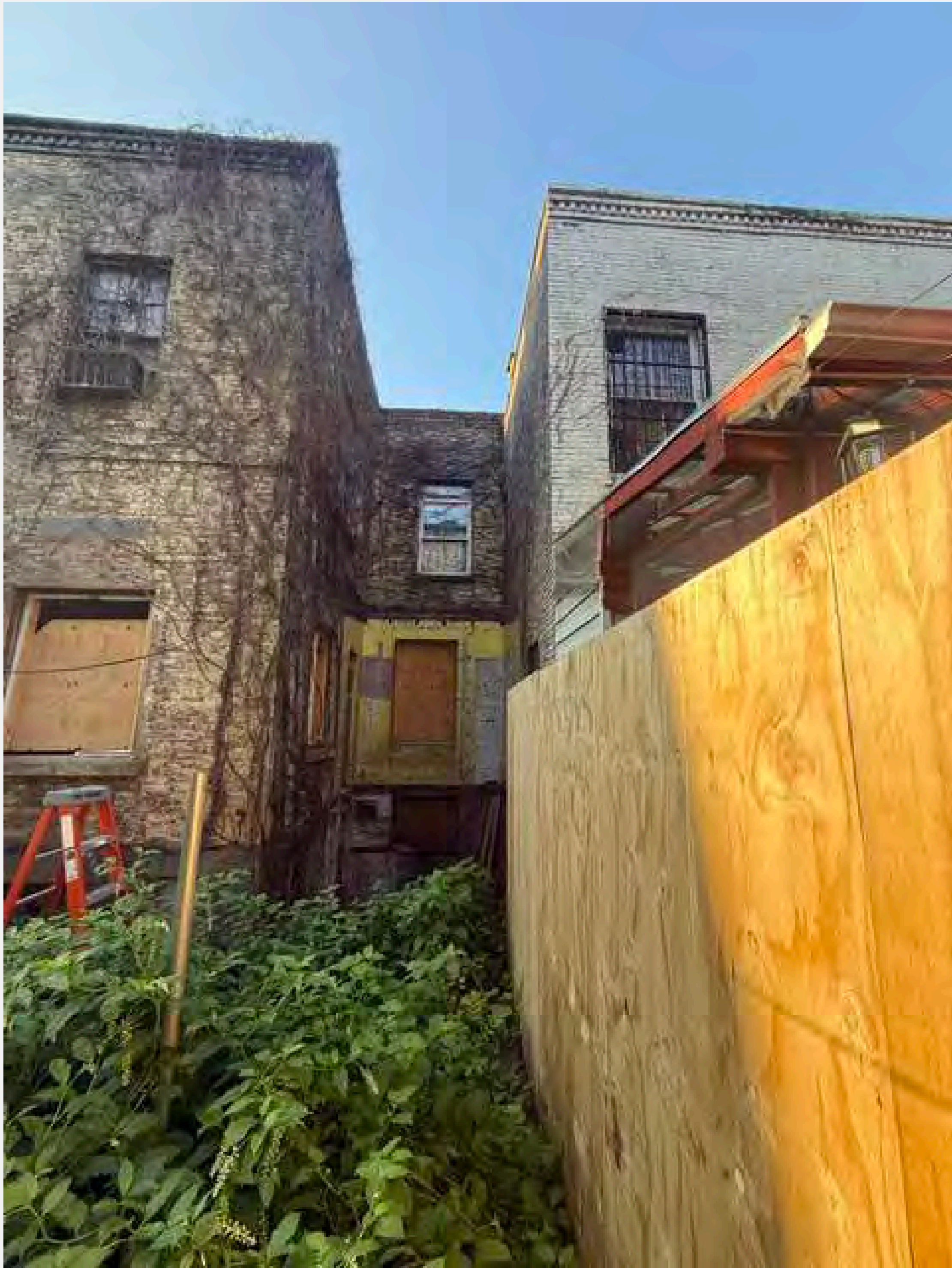
EXISTING REAR FACADE
