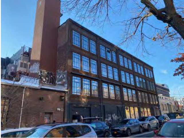
East Facing Facade
