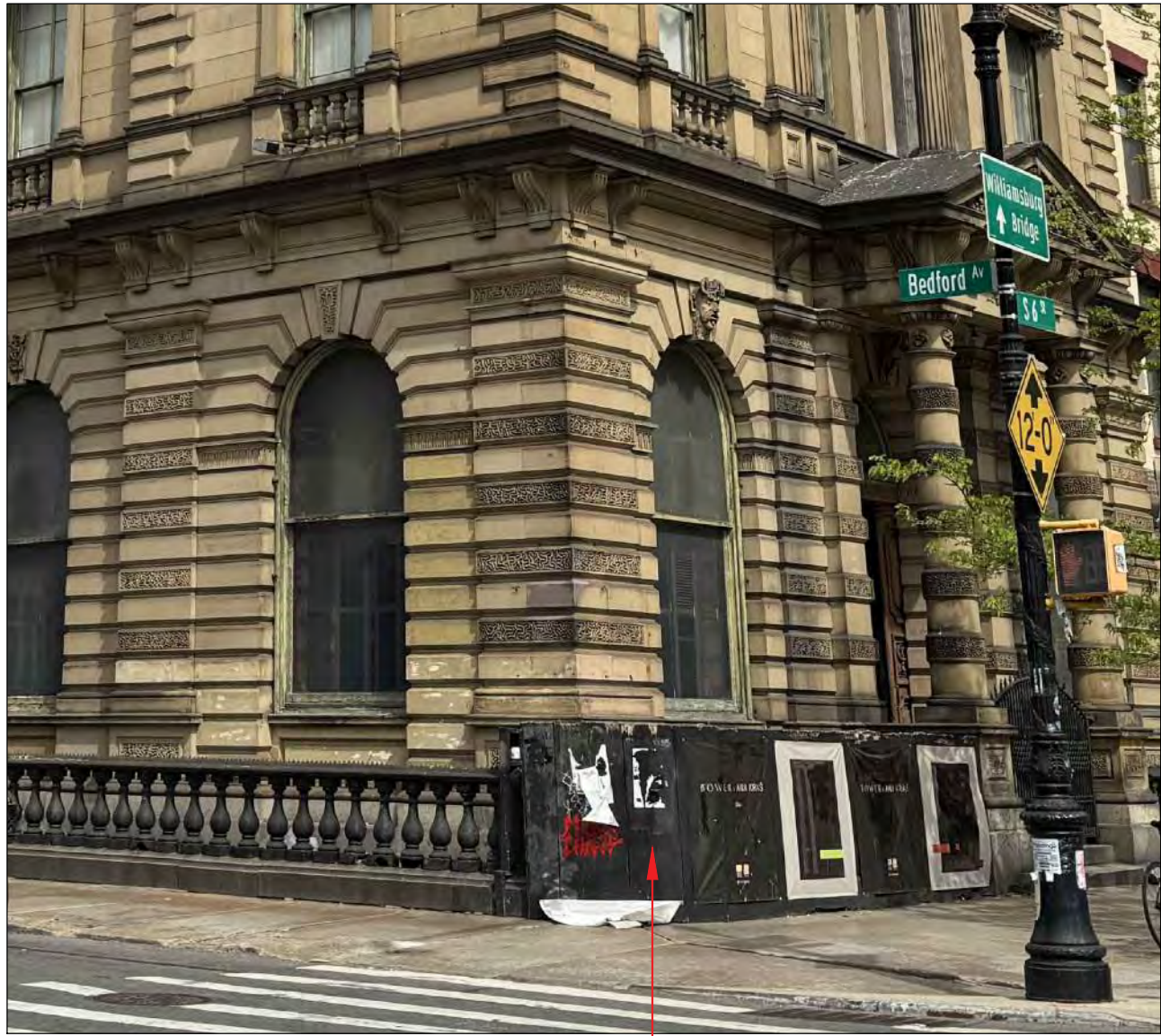
REMOVE TEMPORARY SIGNAGE AND WOOD BARRICADE
