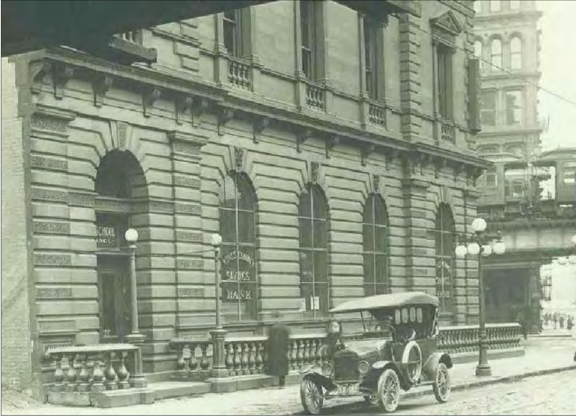
PHOTO 06 CLOSE UP VIEW OF ORIGINAL LAMP POST SOURCE: BROOKLYN PUBLIC LIBRARY YEAR:1920
