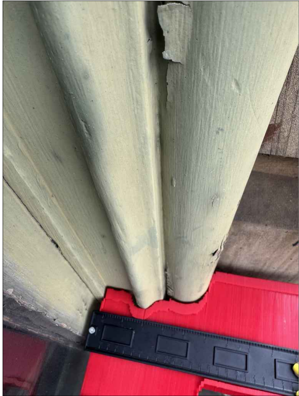
PHOTO 4 CLOSE-UP VIEW AT EXTERIOR WOOD BRICK MOLD
