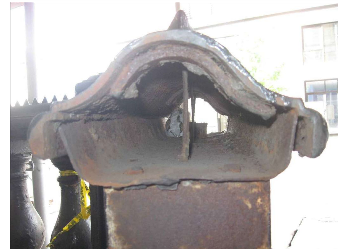
4 EXISTING DETAIL CONNECTION NTS
