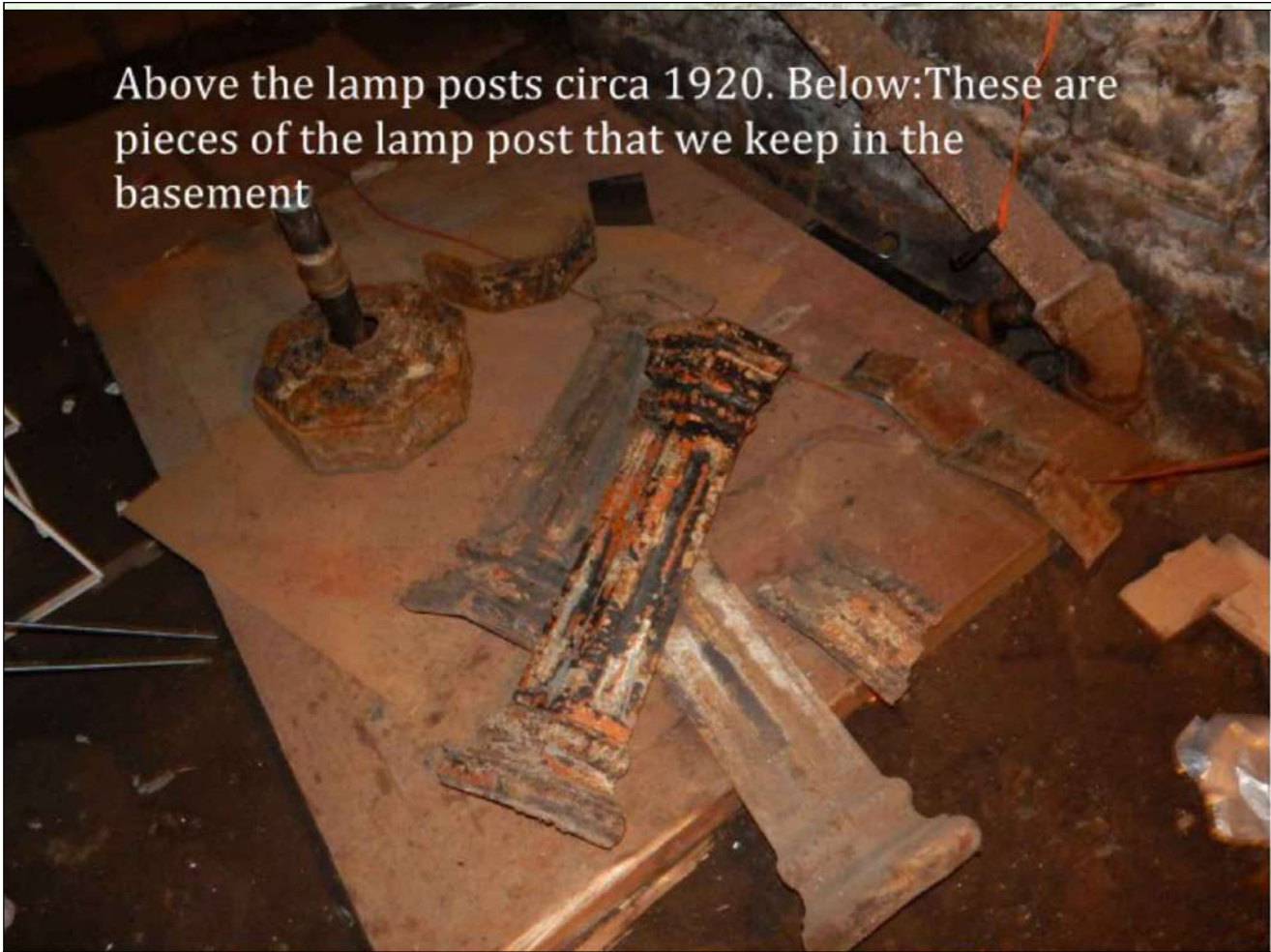
PHOTO 05 CAST IRON LAMP POST PARTS SOURCE: BUILDING OWNER
