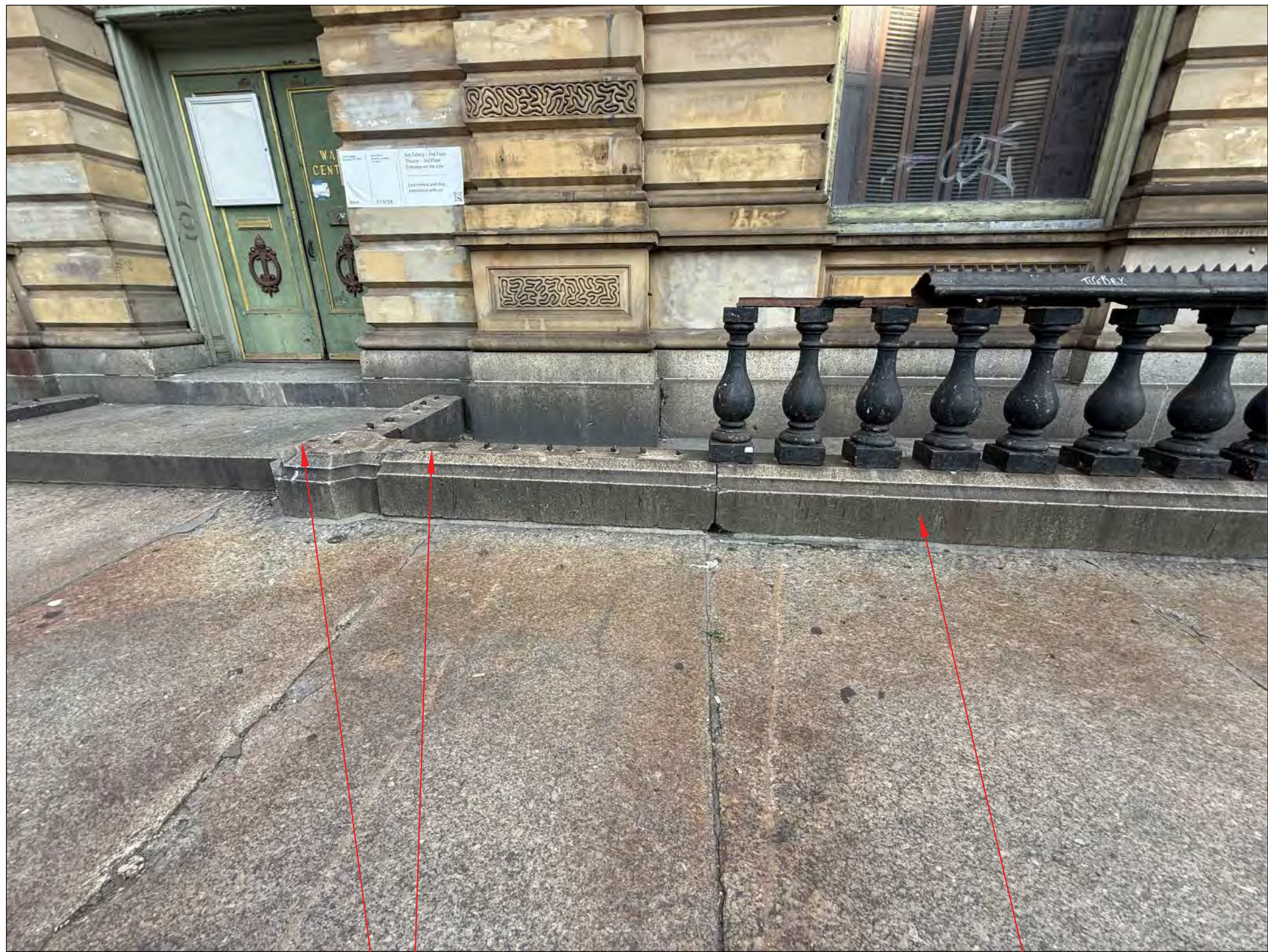
PHOTO 10 AT SIDE BUILDING ENTRANCE FACING WEST
