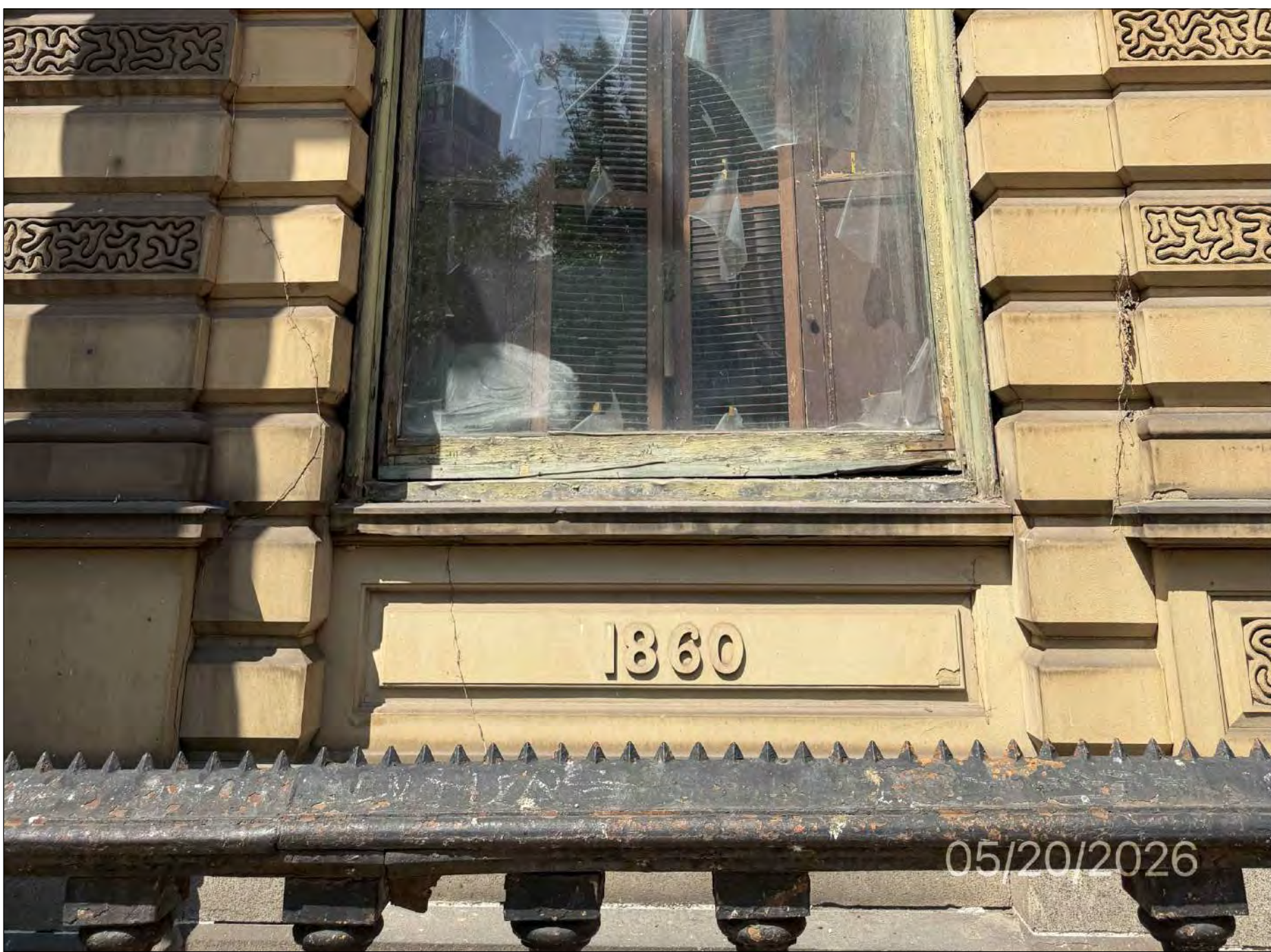
PHOTO 5 CLOSE-UP VIEW AT WINDOWSILL (SOUTH FACING BROADWAY)
