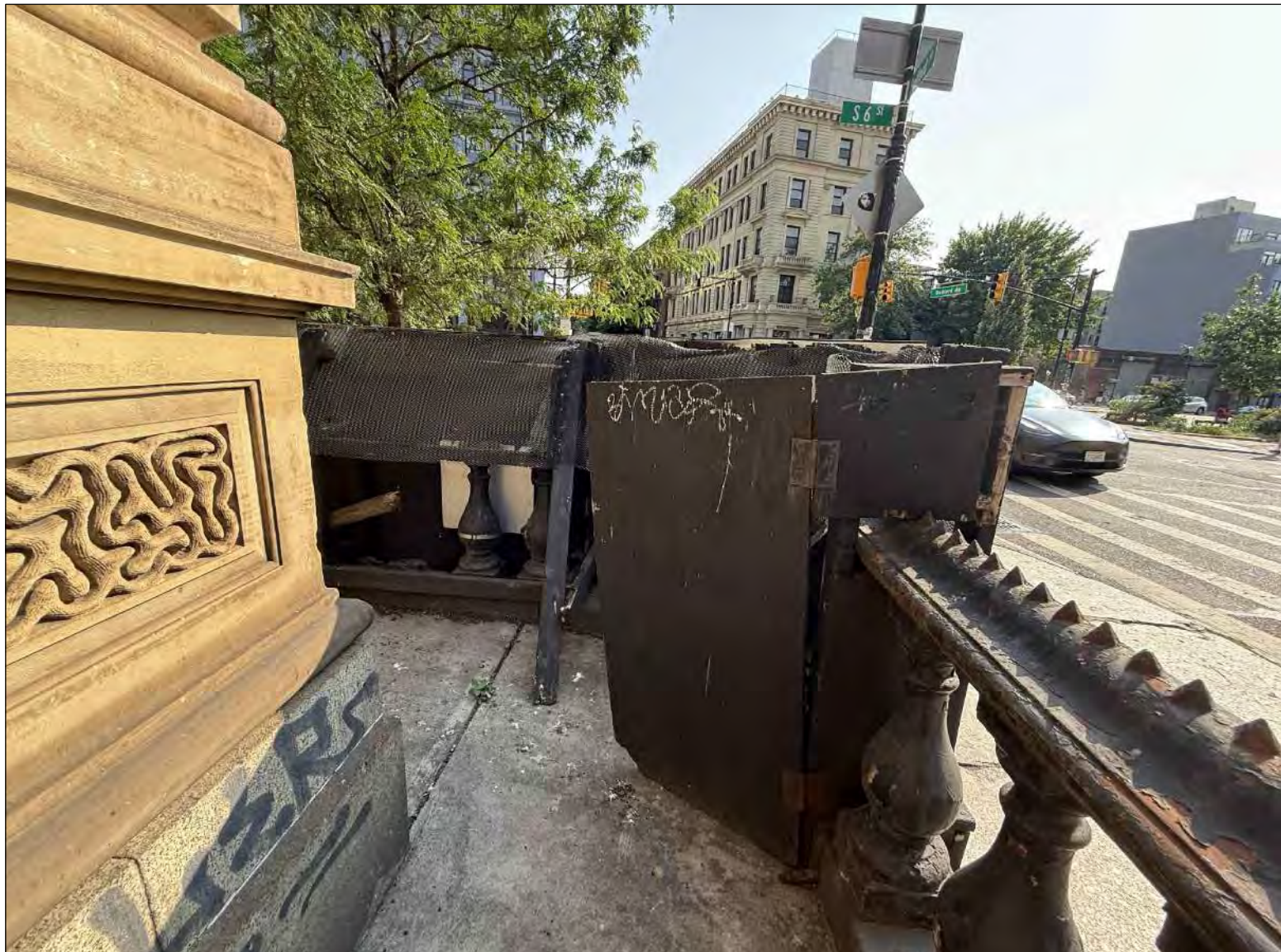
PHOTO 12 PRESENT DAY PHOTO OF TEMPORARY SIGNAGE AND WOOD BARRICADE
