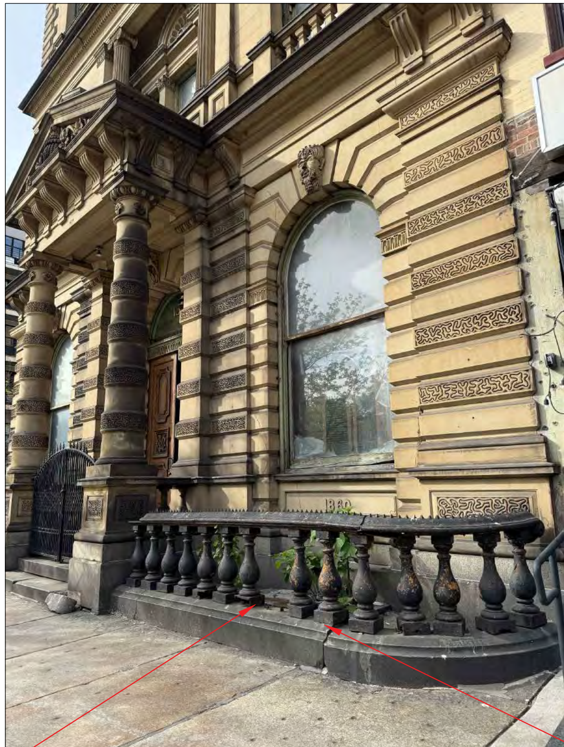
INSTALL REFURBISHED OR RESTORED MISSING CAST IRON BALLUSTERS AND RAILING ON EXISTING OR NEW STONE CURBS.CLEAN, REPAIR AND FILL IN CRACKED STONE AT EXISTING BALLUSTER CURB
