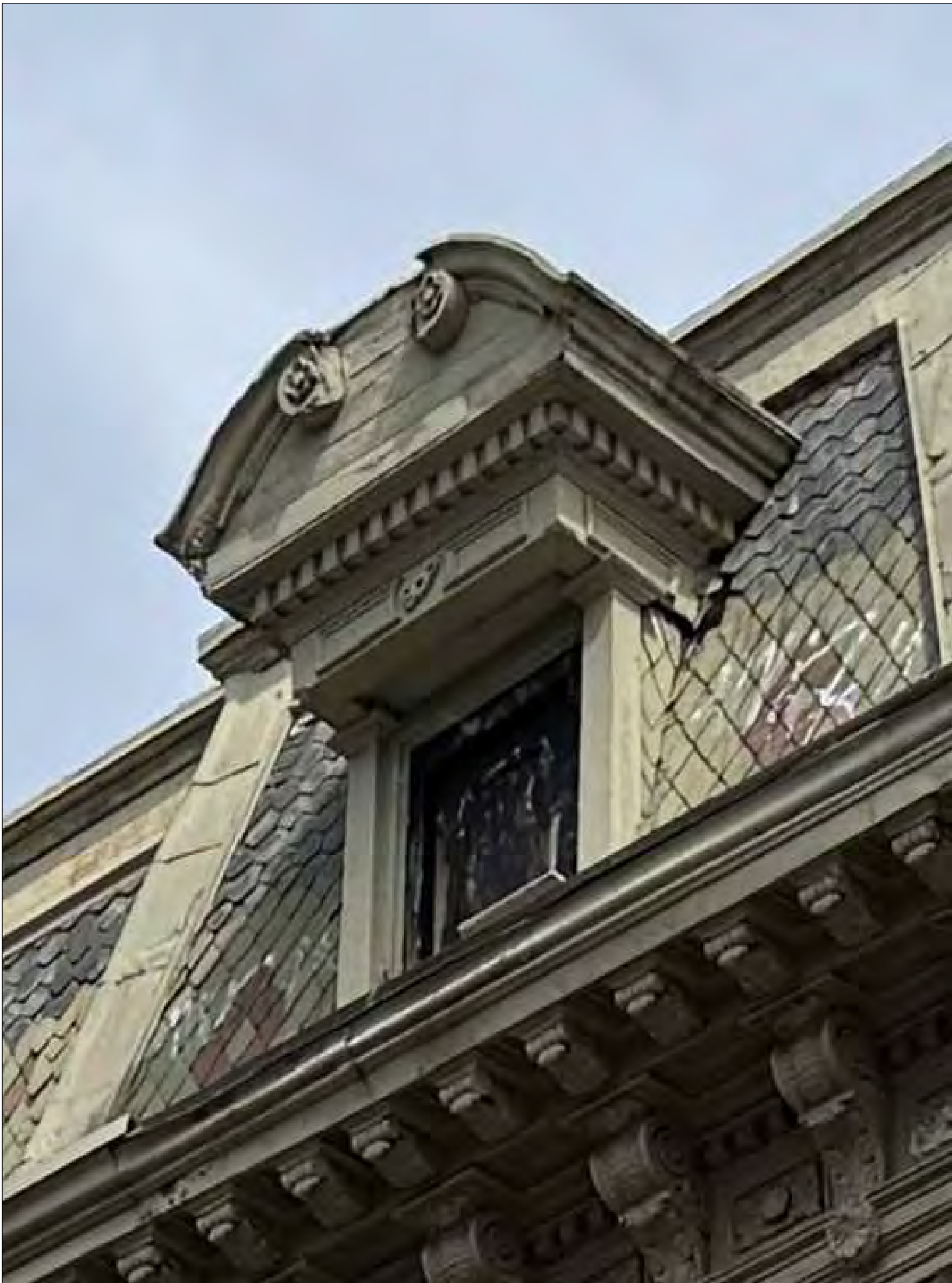
PHOTO 8 VIEW AT ATTIC FLOOR WINDOW FACING BEDFORD AVE
