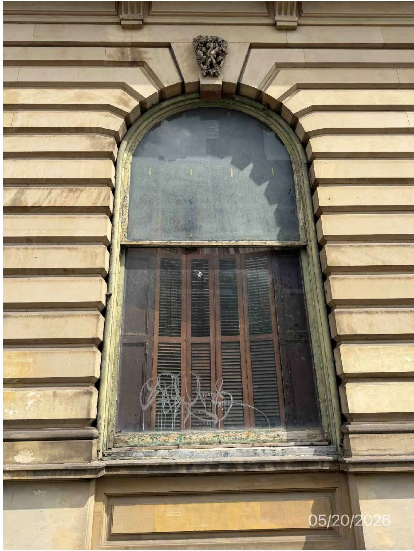
PHOTO 3 VIEW AT FIRST FLOOR WINDOW FACING BEDFORD AVENUE
