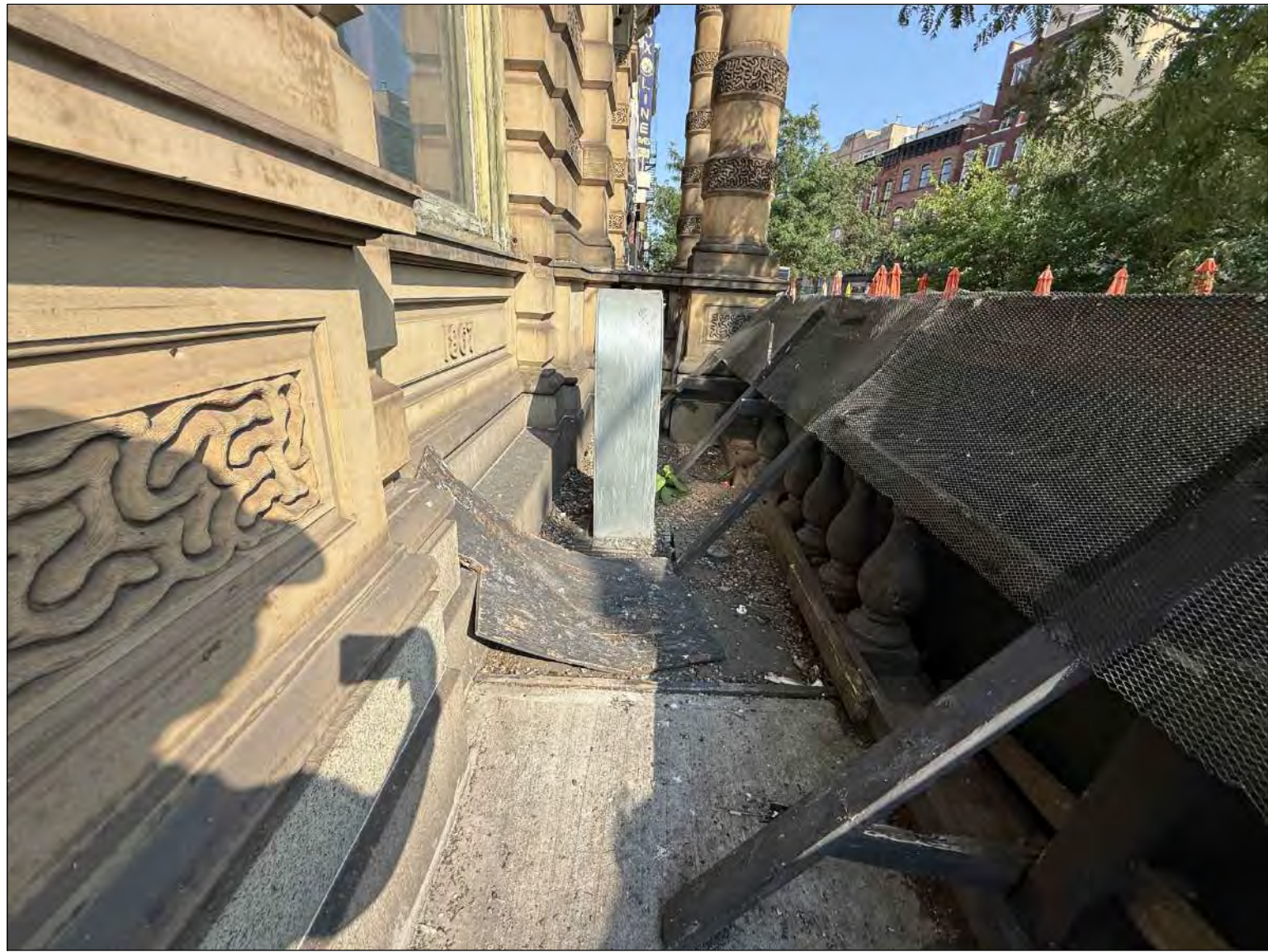
PHOTO 13 PRESENT DAY PHOTO AT EXISTING FRESH AIR DUCT AT EXISTING WINDOW WELL
