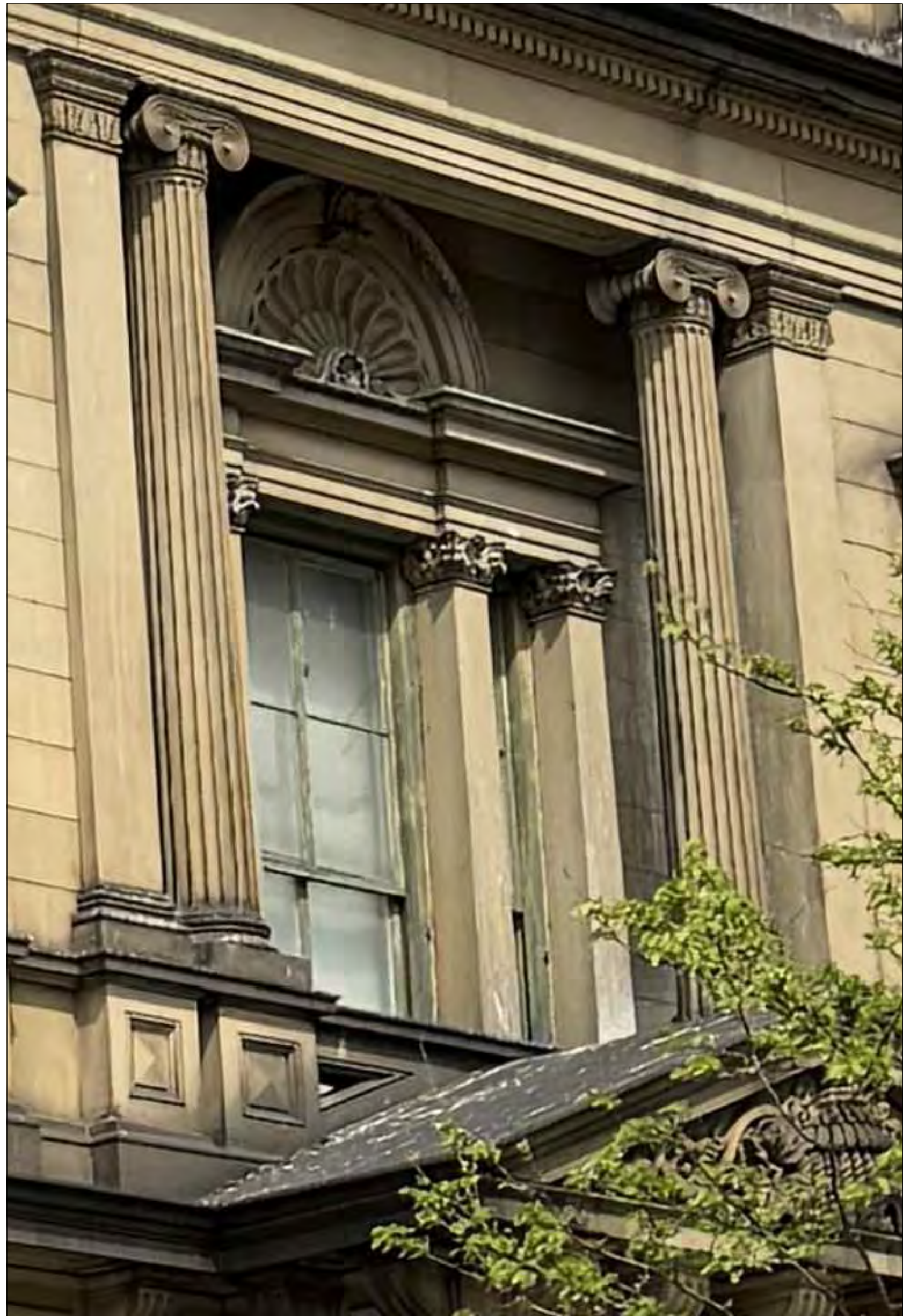
PHOTO 7 VIEW AT SECOND FLOOR WINDOW FACING BROADWAY
