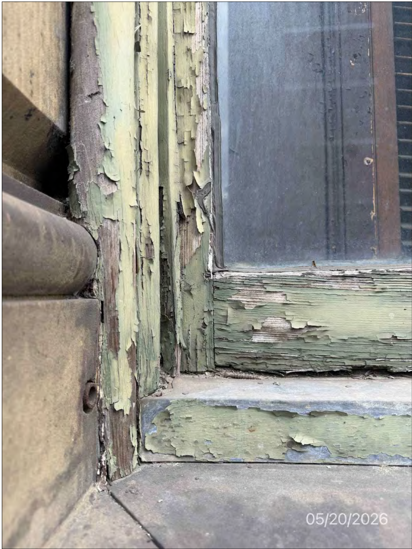
PHOTO 6 CLOSE UP VIEW AT EXG WINDOWSILL AND BRICK MOLD
