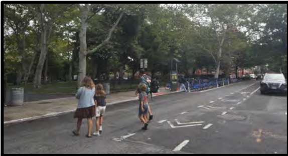
New Neckdown & Stop Sign (Similar treatment at North Henry & Nassau)
