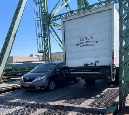
Typical Condition with Traffic on the Bridge
