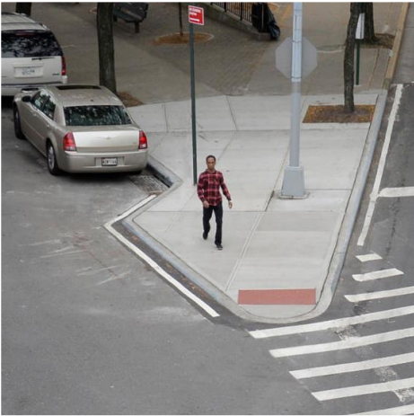
Concrete Sidewalk Extensions
