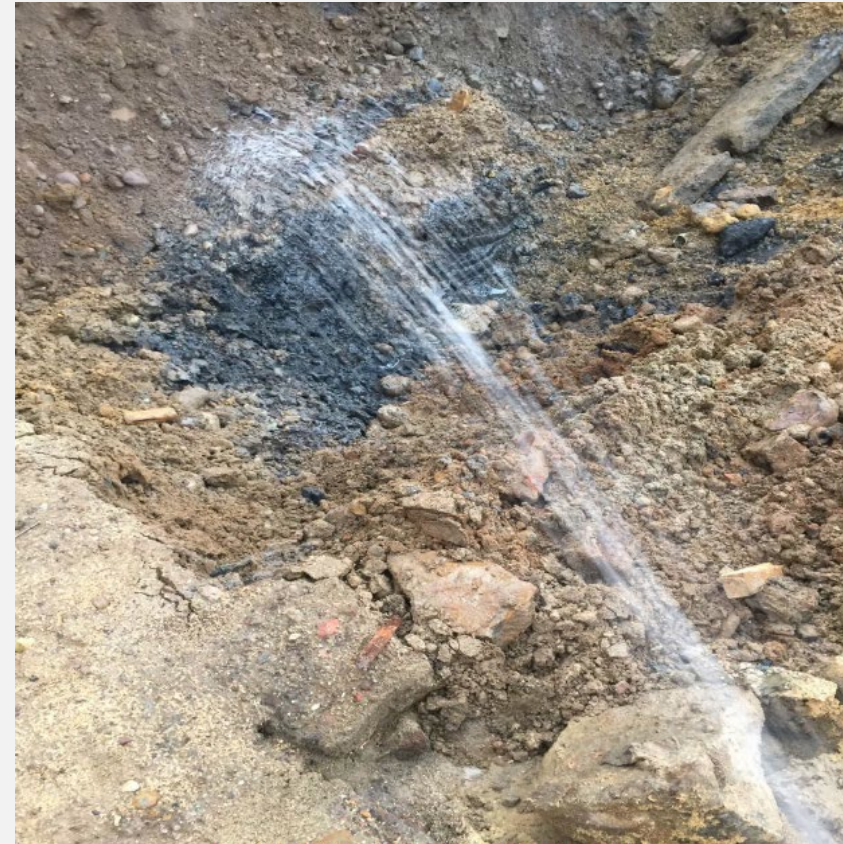
Applied L-10 odor suppression to control odors
