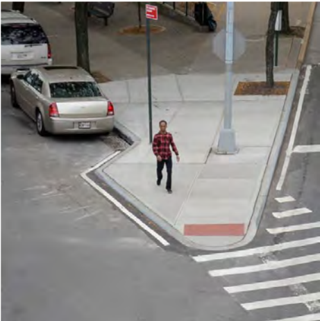
Concrete Sidewalk Extensions
