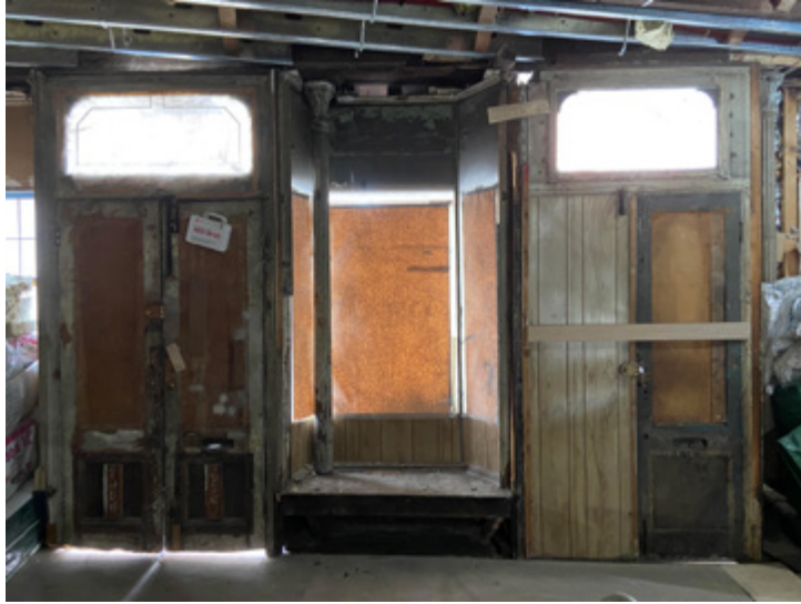
INTERIOR FACE OF EXISTING STOREFRONT
