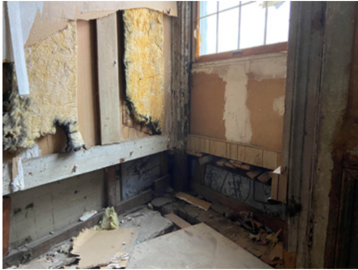
INTERIOR FACE OF CORNER CONDITION
