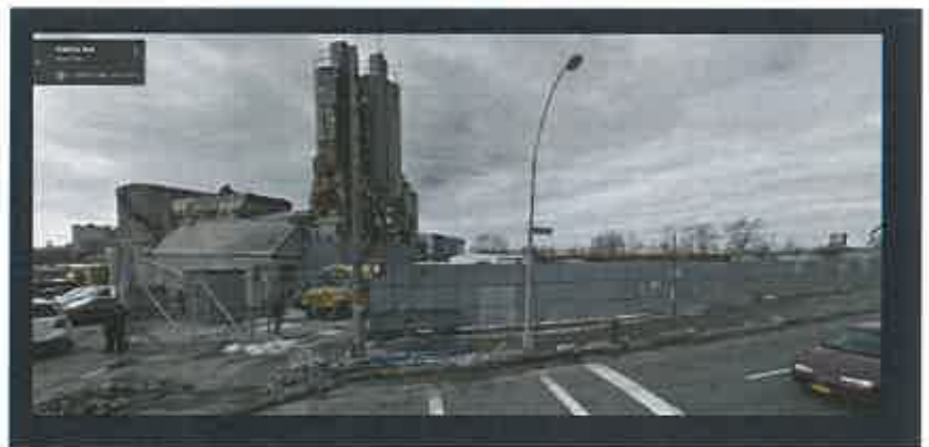
Before (right) and after (below) CubeSmart 2990 Cropsey Ave.
