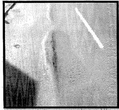
Many of CB#1's streets are riddled with roadway problems, such as hummocks, resulting from the constant heavy truck traffic. The asphalt becomes rutted and pushed up creating vehicular, pedestrian and cycling hazards. DOT must address this issue ASAP.
