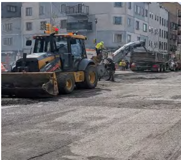
Asphalt milling at Lee Avenue and Wallabout Street intersection.
