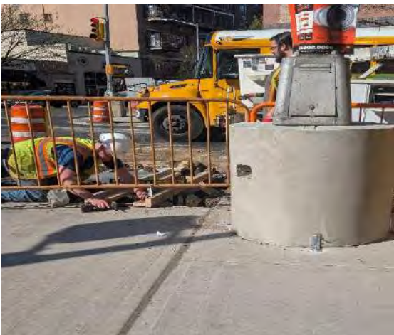
APS and light pole foundation at Lee Avenue and Wallabout Street intersection.
