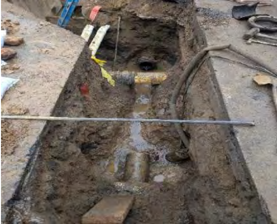
Water Main Installation at Wallabout Street and Lee Avenue.
