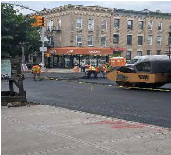
Asphalt Pavement at 60 th Street and 7 th Avenue intersection.
