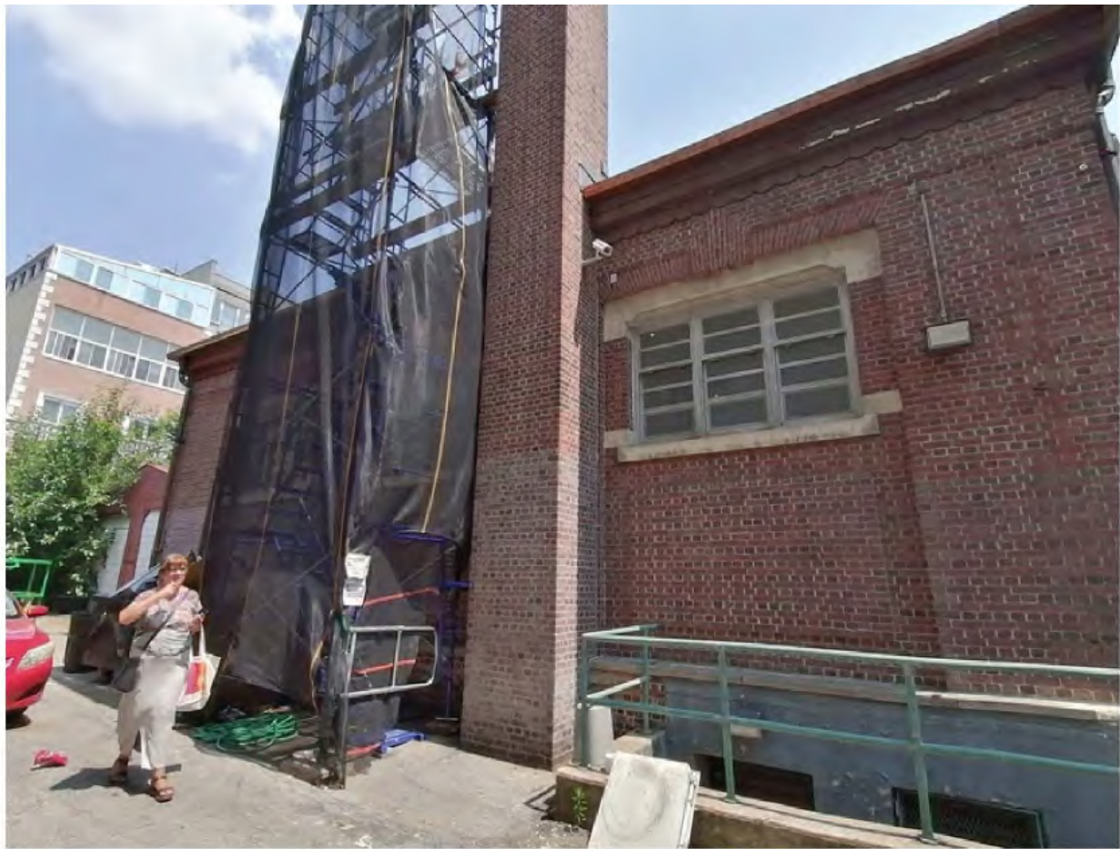
PHOTO 7: EXISTING VIEW OF EAST ELEVATION
