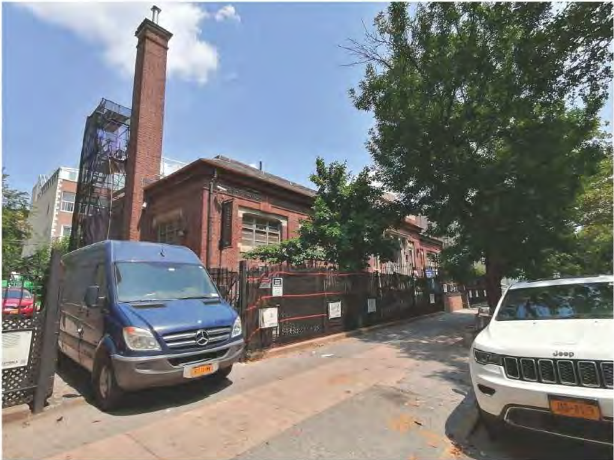
PHOTO 2: EXISTING VIEW OF ENTRANCE AT PARKING AREA
