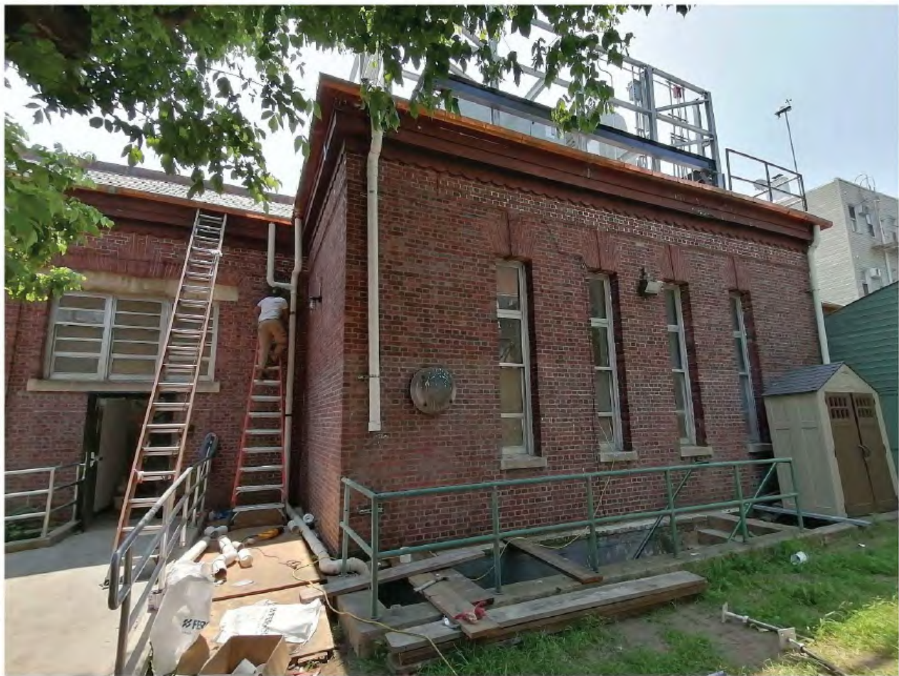
PHOTO 6: EXISTING VIEW OF REAR / NORTH ELEVATION
