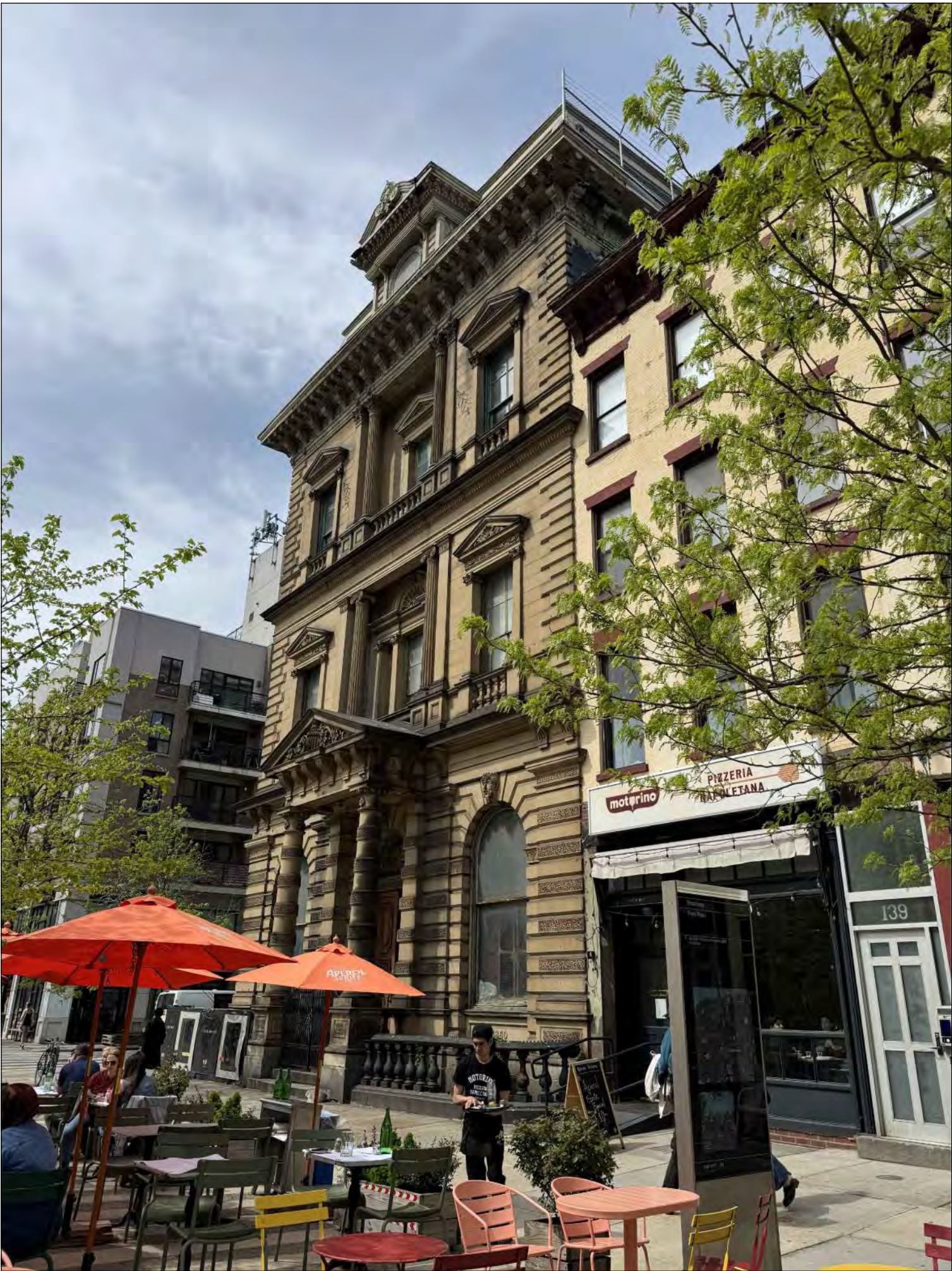
PHOTO 6 PRESENT DAY PHOTO AT BROADWAY - SOUTH FACING PRIMARY ELEVATION
