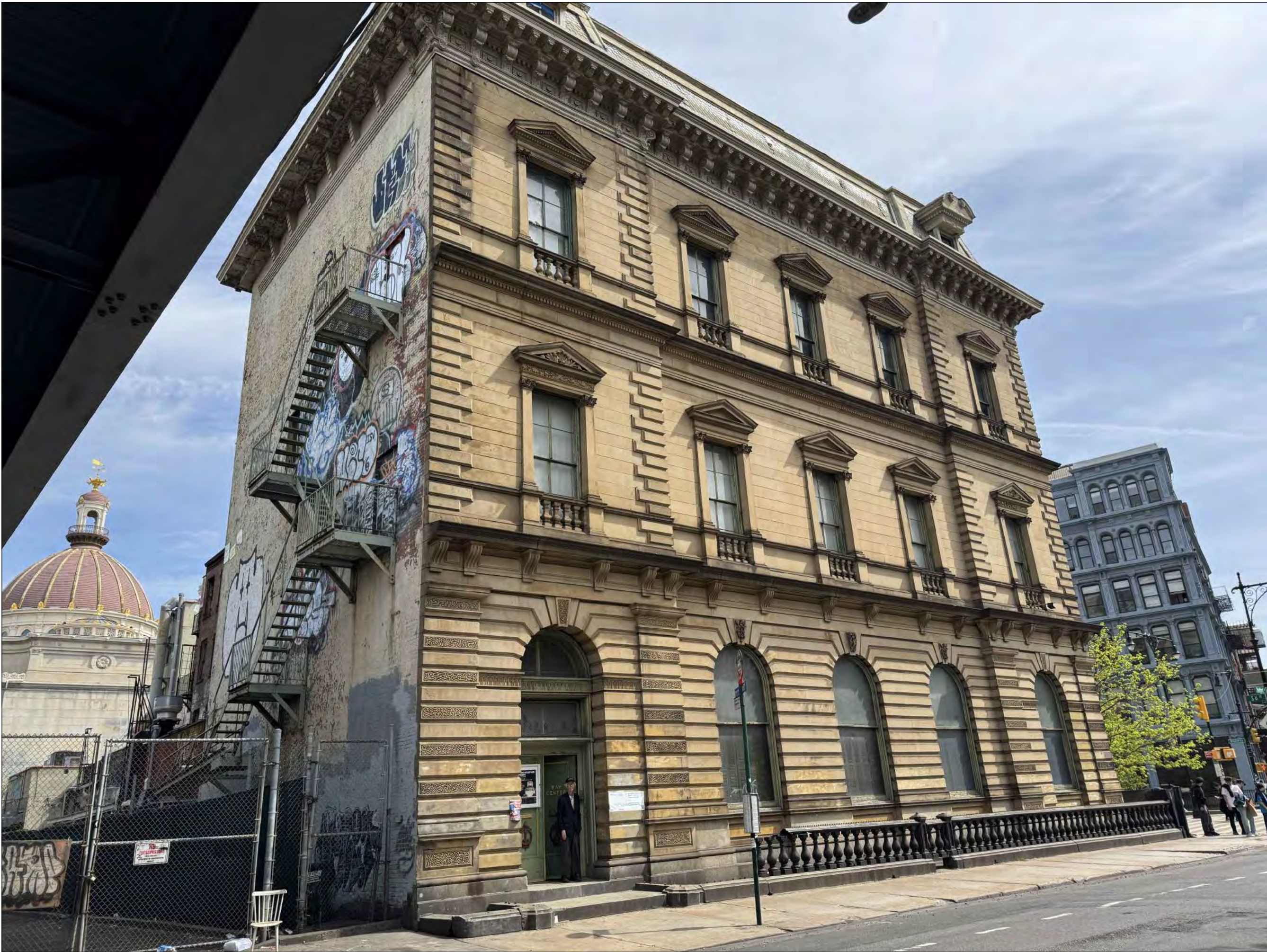
PHOTO 5 PRESENT DAY PHOTO AT BEDFORD AVENUE - WEST FACING PRIMARY ELEVATION
