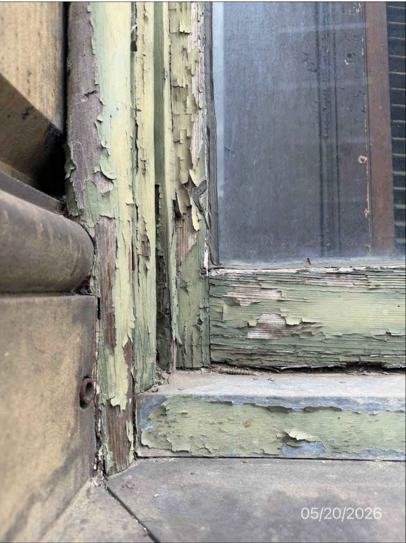
PHOTO 13 CLOSE UP VIEW AT EXG WINDOWSILL AND BRICK MOLD
