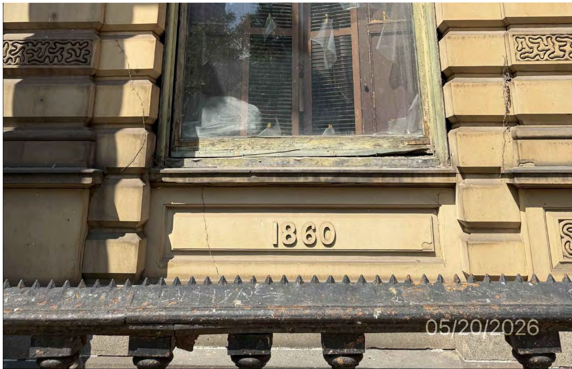
PHOTO 12 CLOSE-UP VIEW AT WINDOWSILL (SOUTH FACING BROADWAY)
