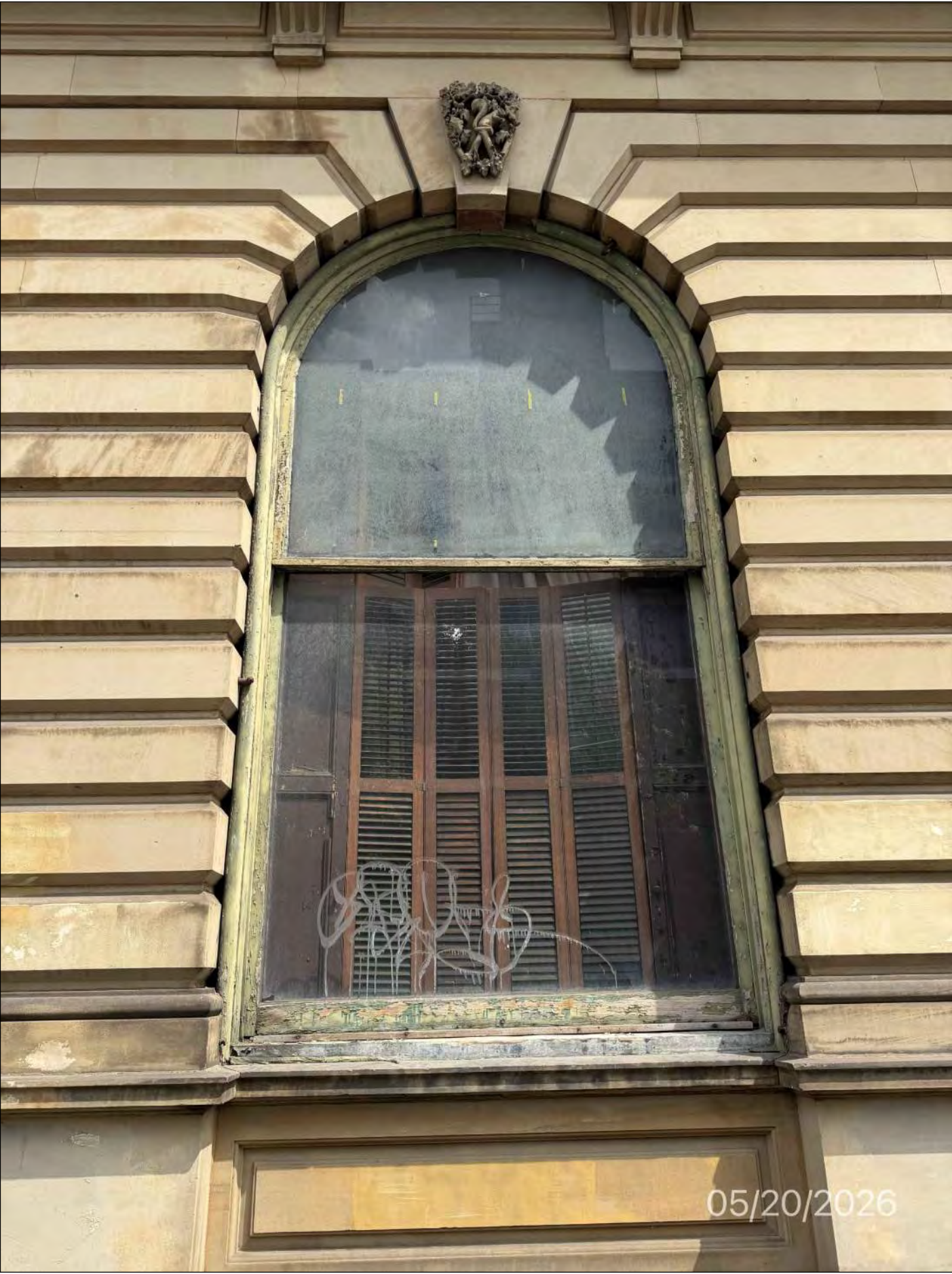
PHOTO 10 VIEW AT FIRST FLOOR WINDOW FACING BEDFORD AVENUE
