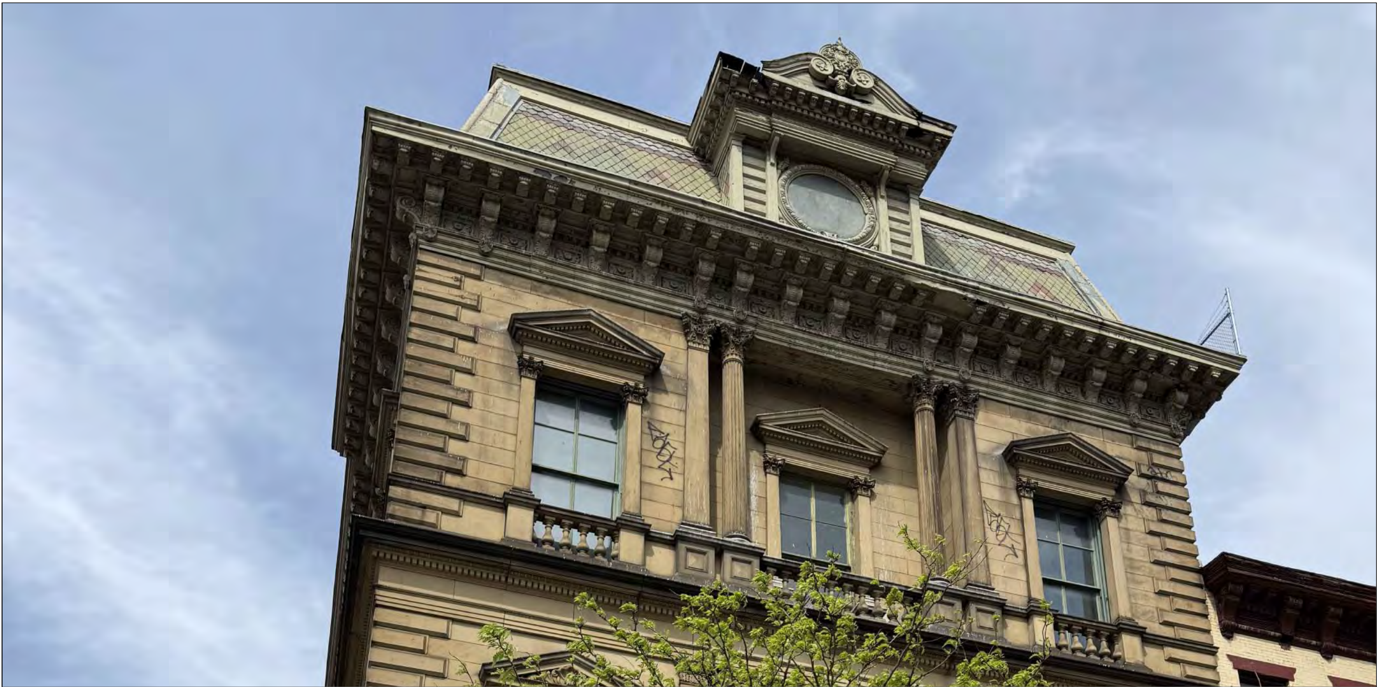
PHOTO 7 PRESENT DAY CLOSE-UP VIEW AT 3RD FLOOR WINDOWS AND CORNICE FACING SOUTH
