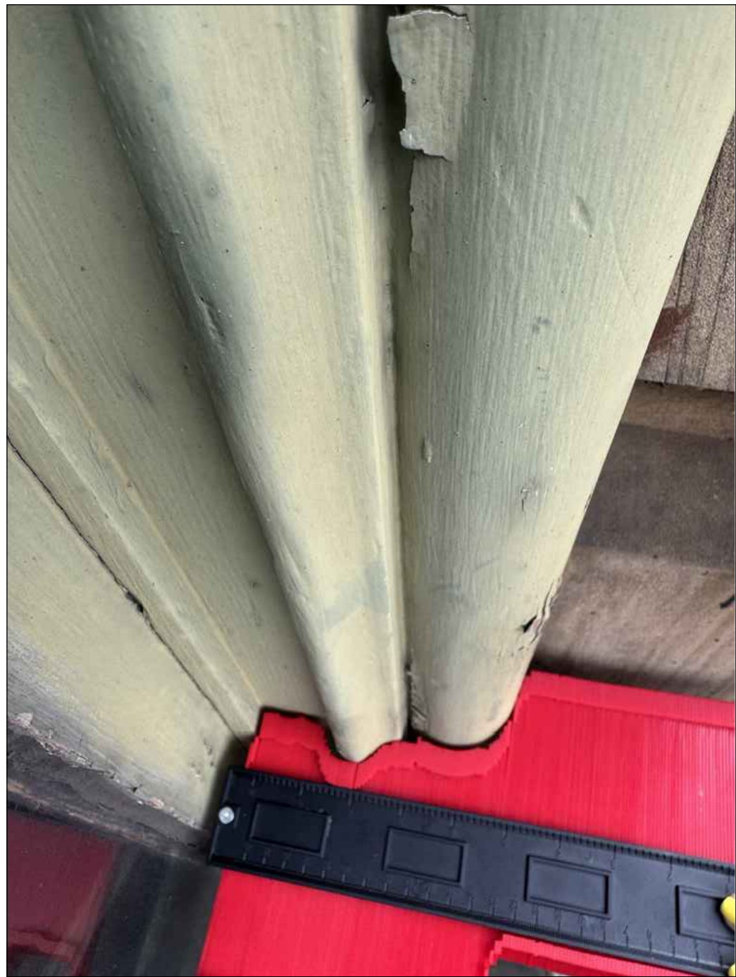
PHOTO 11 CLOSE-UP VIEW AT EXTERIOR WOOD BRICK MOLD
