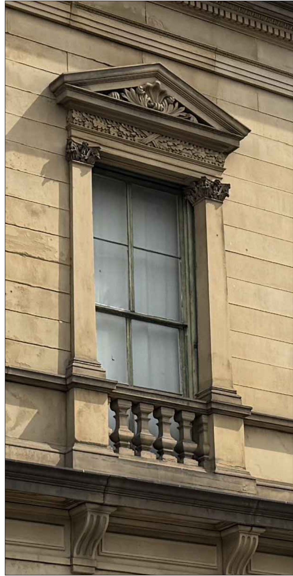
PHOTO 8 VIEW AT 2ND FLOOR WINDOW AT BEDFORD AVENUE
