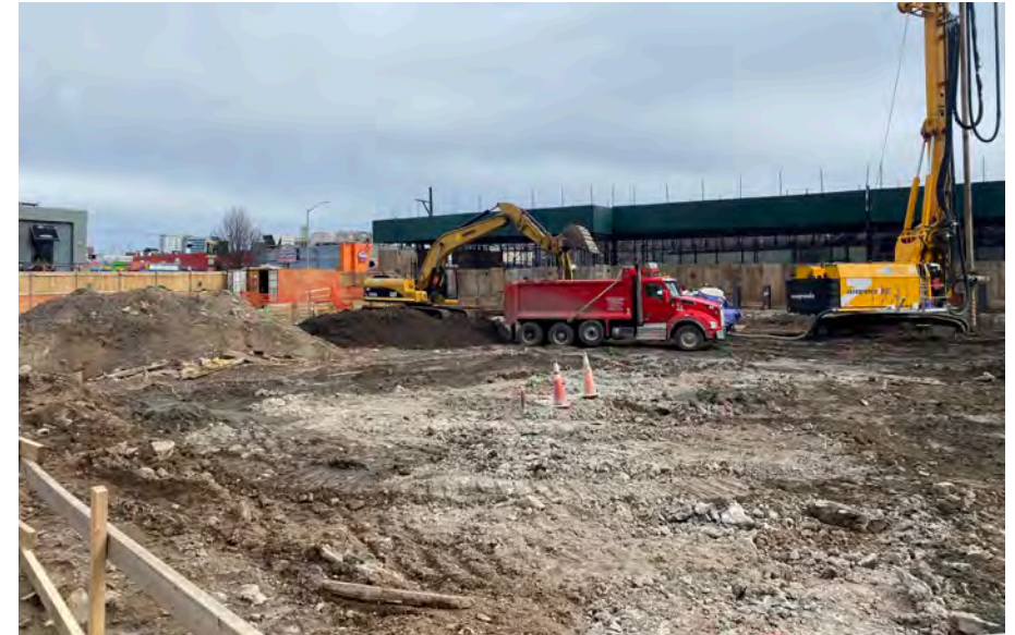
Direct-Load Soil for Off-Site Disposal
