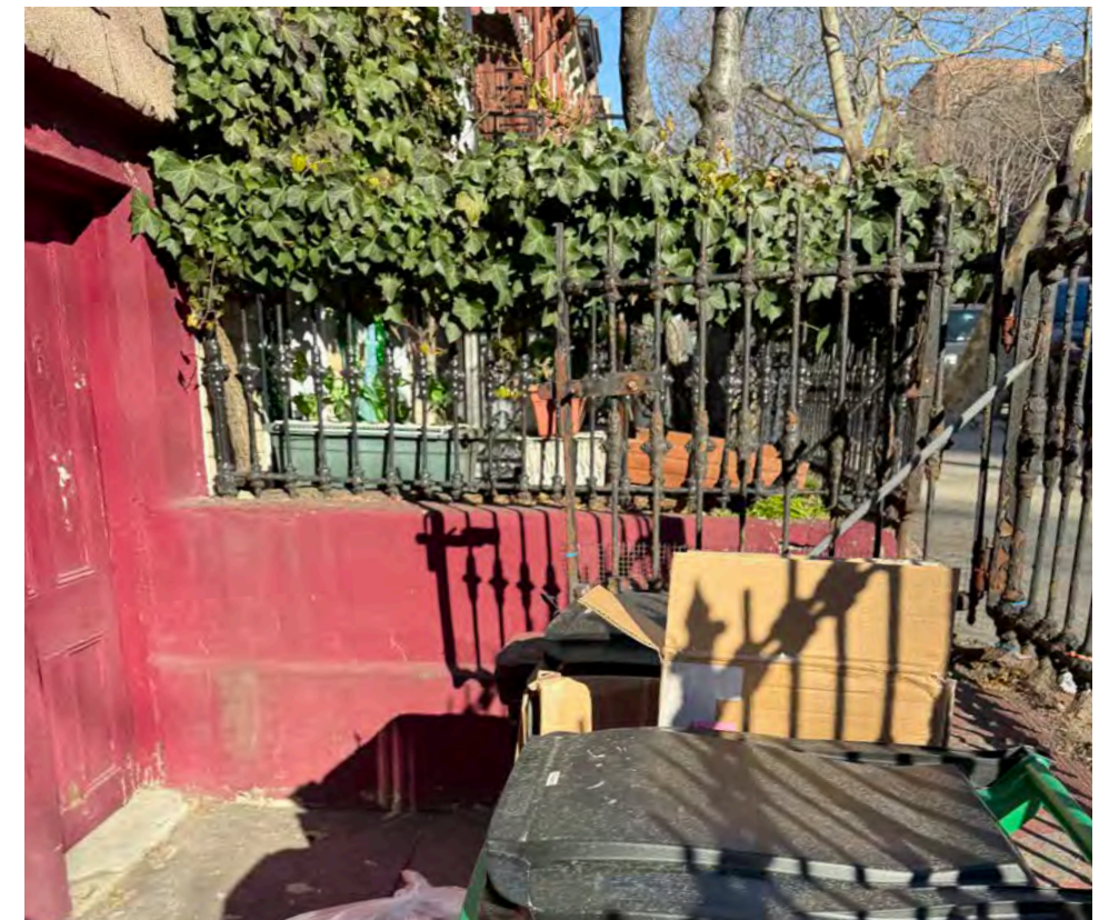
113 NOBLE STREET, EXISTING FRONT AREAWAY IRONWORK
