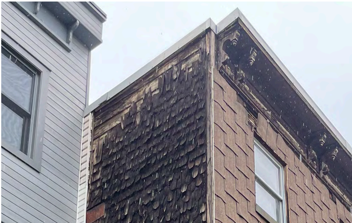
113 NOBLE STREET, EXISTING CLAPBOARD & NOVELTY SHINGLE LAYERS
