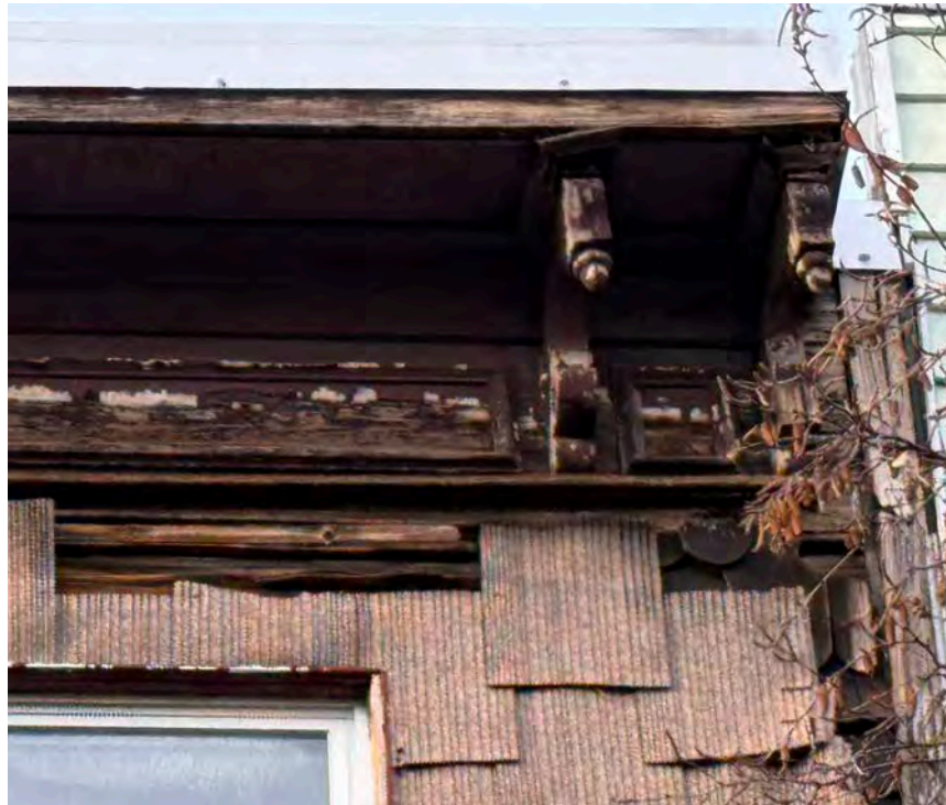
113 NOBLE STREET, EXISTING CLAPBOARD, NOVELTY SHINGLE & ASPHALT SHINGLE LAYERS
