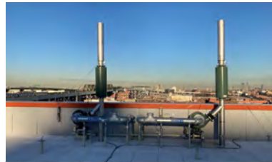
Roof-Mounted Fans and Exhaust
