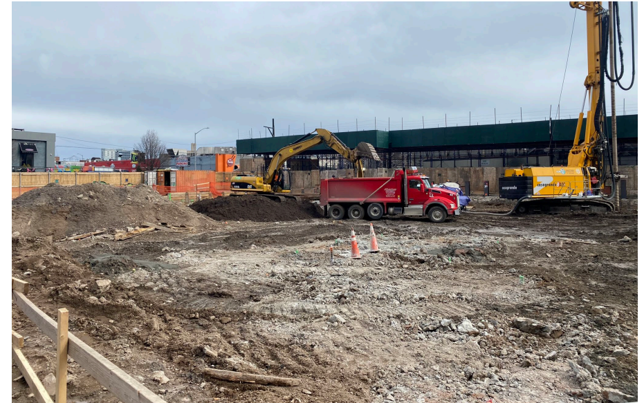
Direct-Load Soil for Off-Site Disposal
