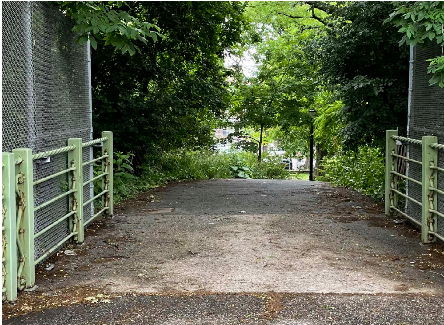
1 - view of top of ramp connection to bridge
