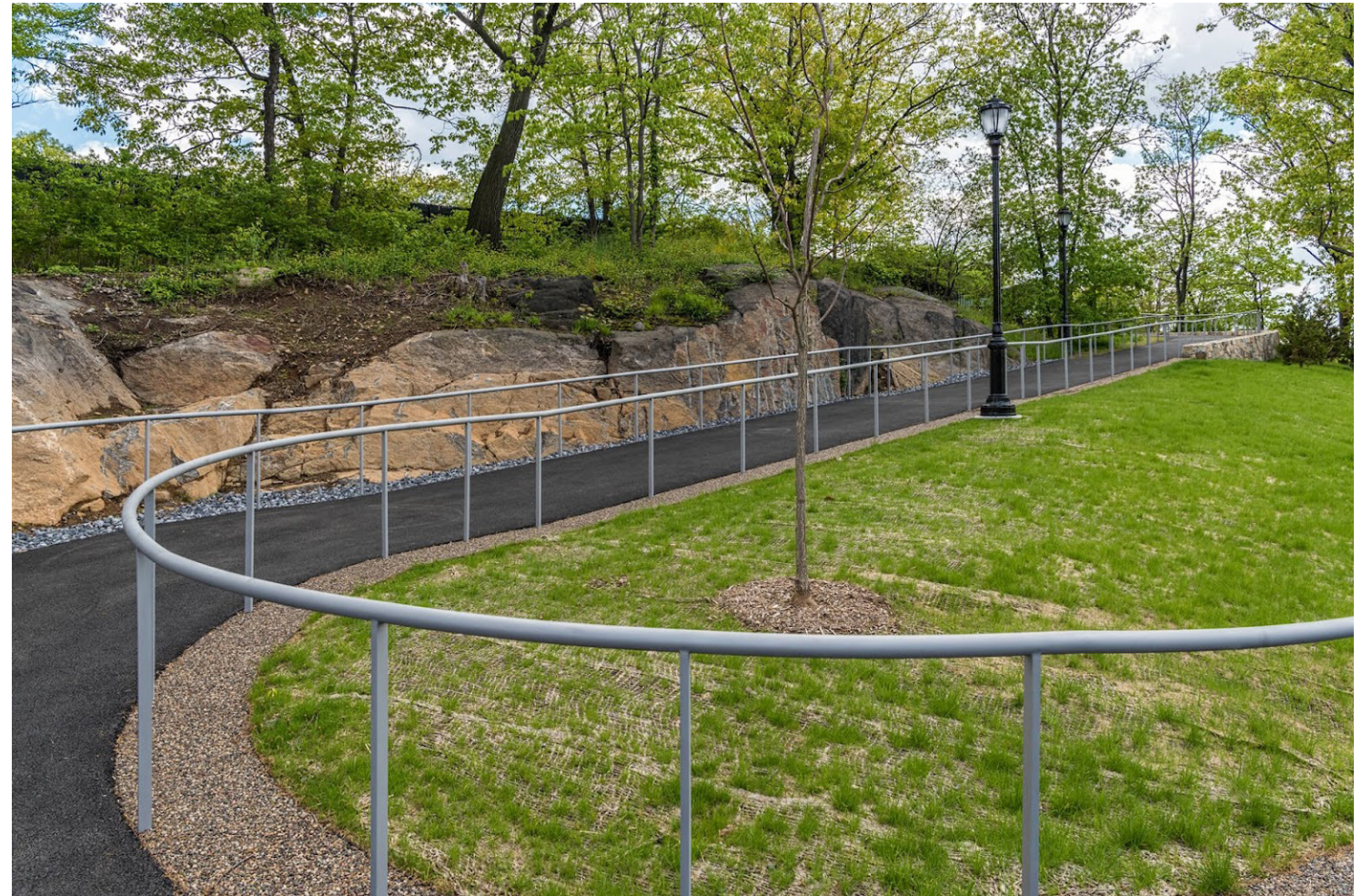
3 - Middle of ramp
