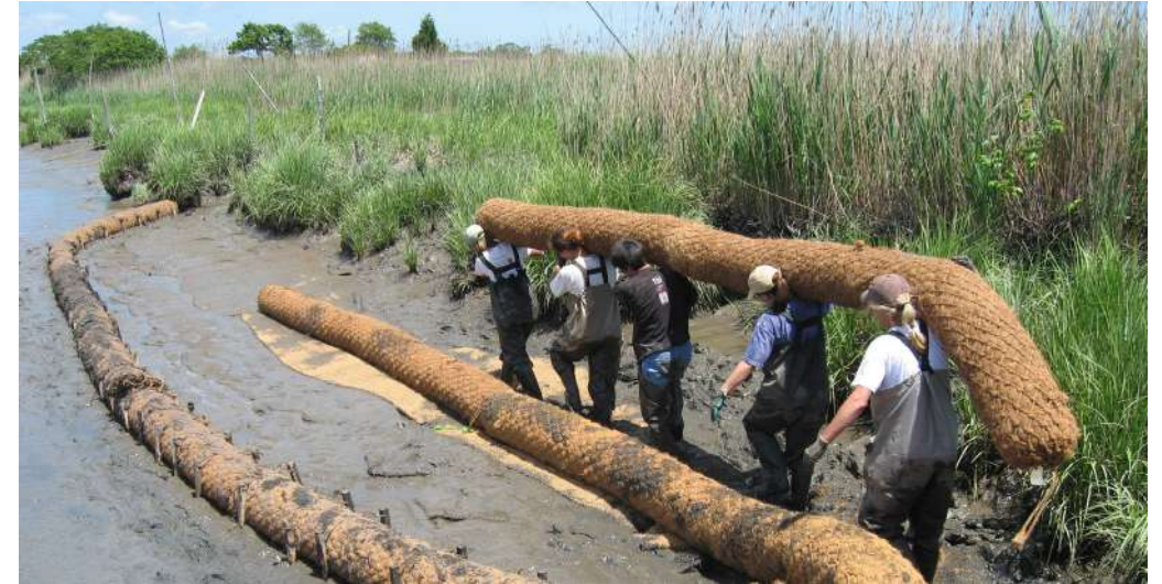
Installation of coir logs to stabilize eroding shoreline photo credit: Mike Shanahan, CoastalResilience.org
