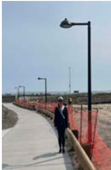
Davit-fixtured 12' Pedestrian light pole
