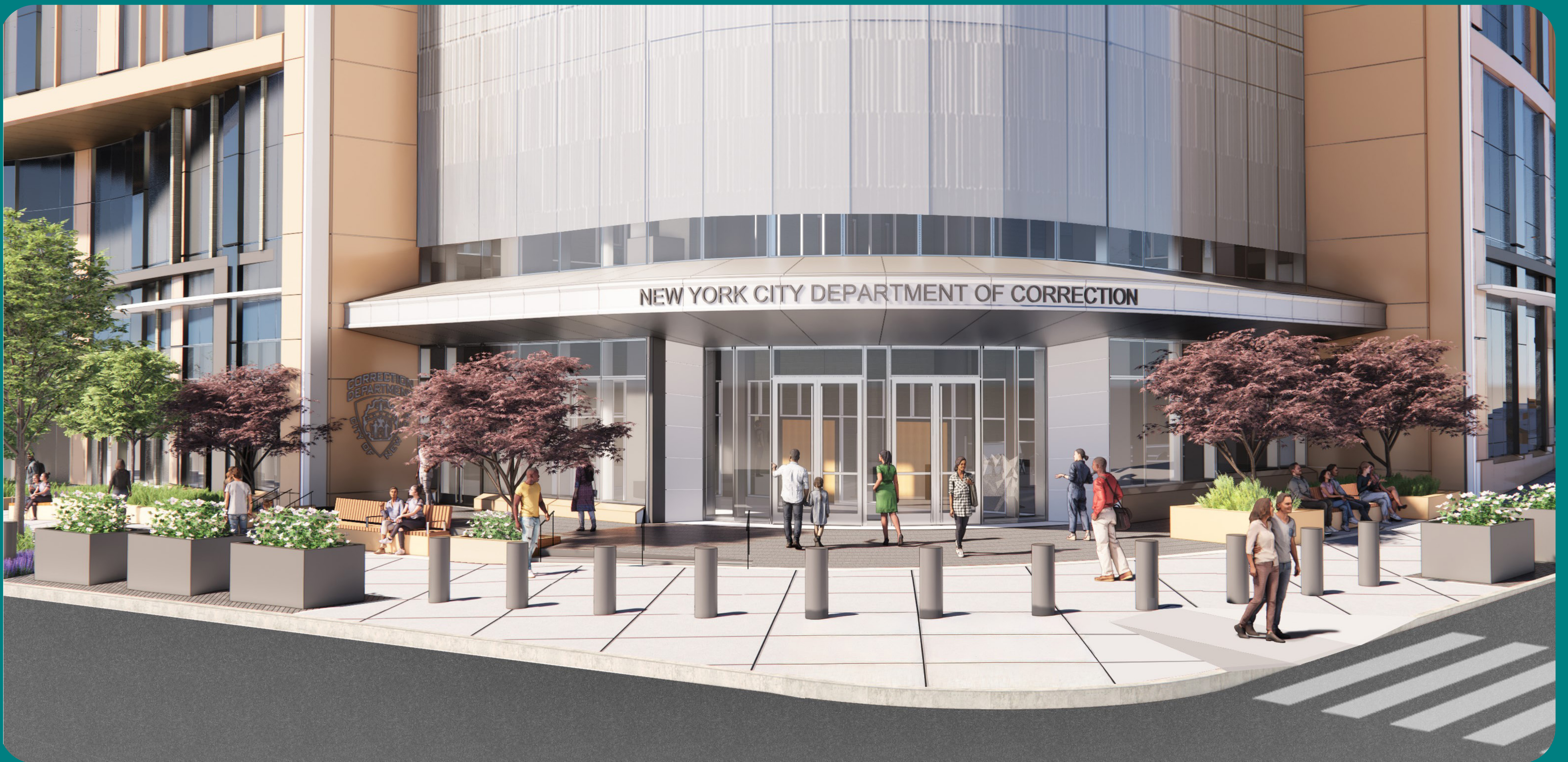
PUBLIC LOBBY ENTRANCE VIEW AT EAST 142ND STREET & SOUTHERN BOULEVARD
