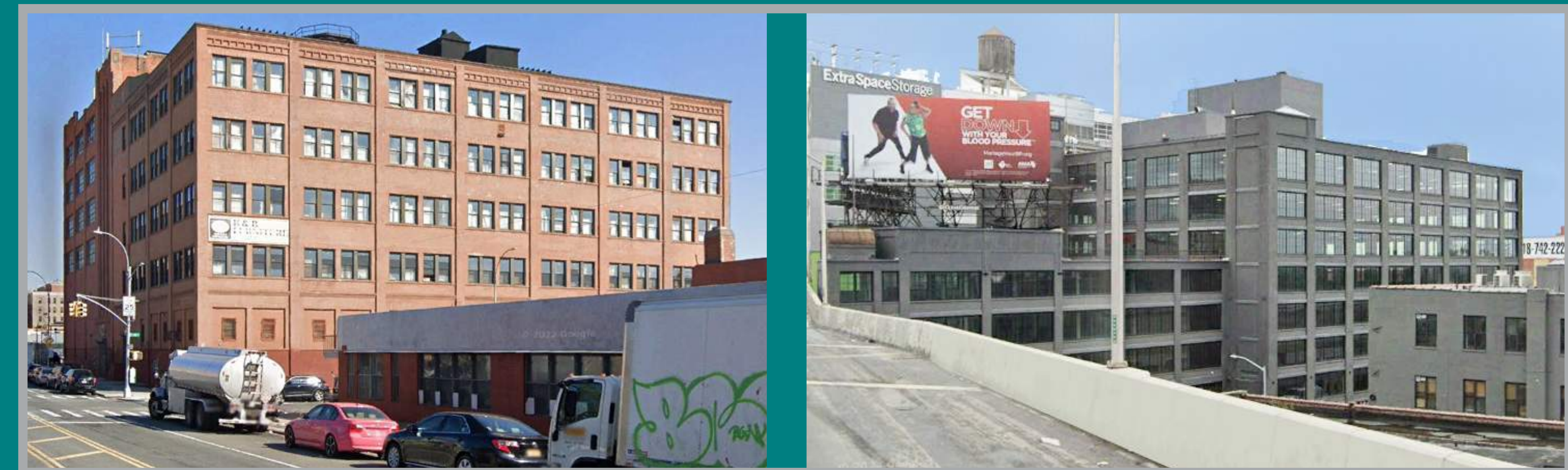
INDUSTRIAL BUILDINGS ADJACENT TO THE SITE EDIFICIOS INDUSTRIALES ADYACENTES A LA OBRA
