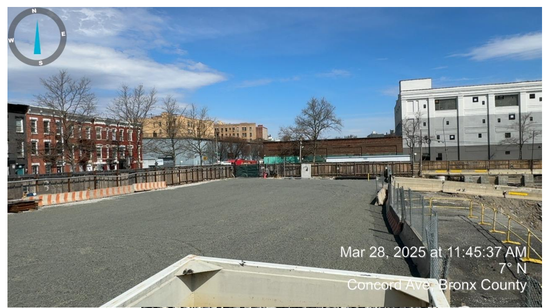
Photos of Tracking Pad installed for Dust & Sediment Control
