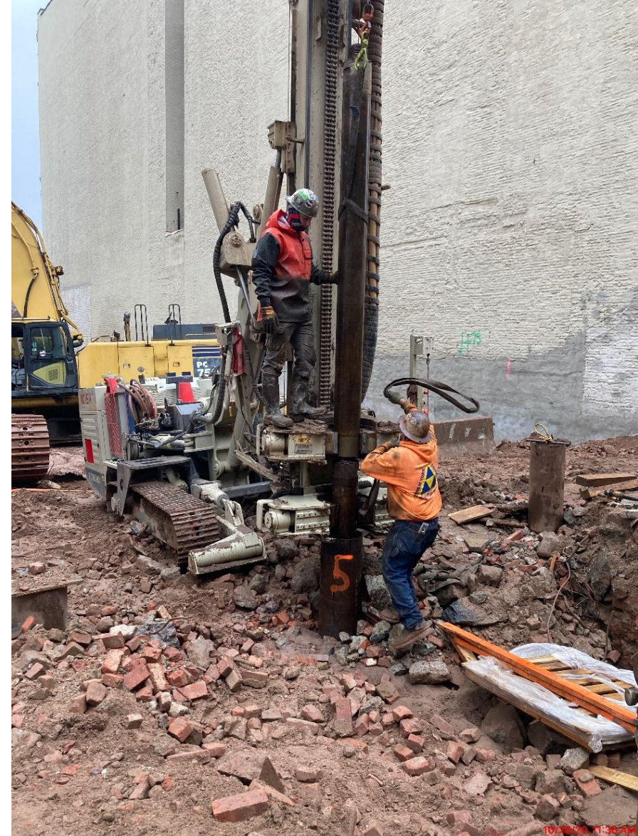
Typical Representation of SOE Installation (Not Bronx Project)
