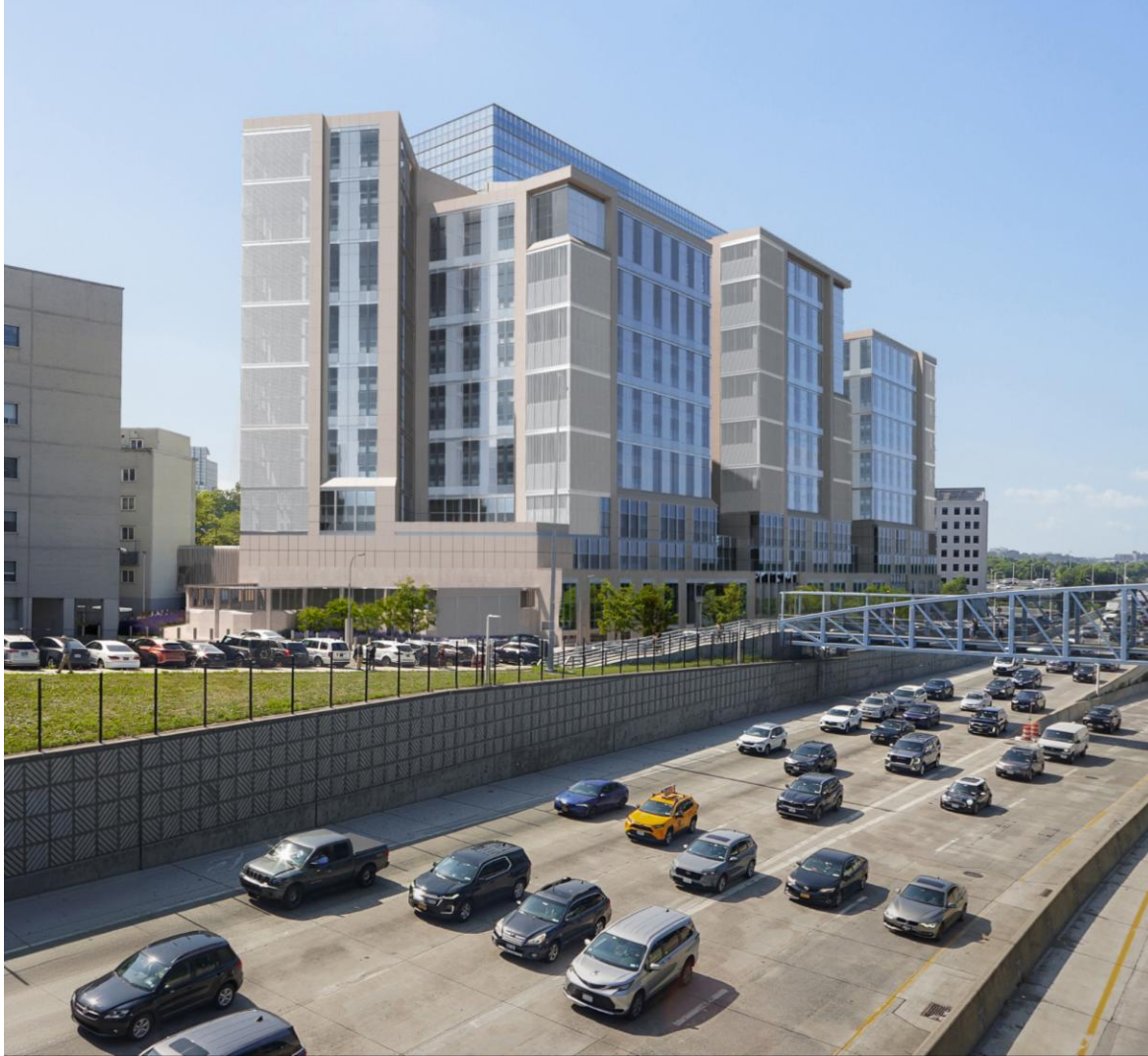
F – View from Hoover Avenue Bridge
