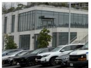
Municipal Parking Garage
