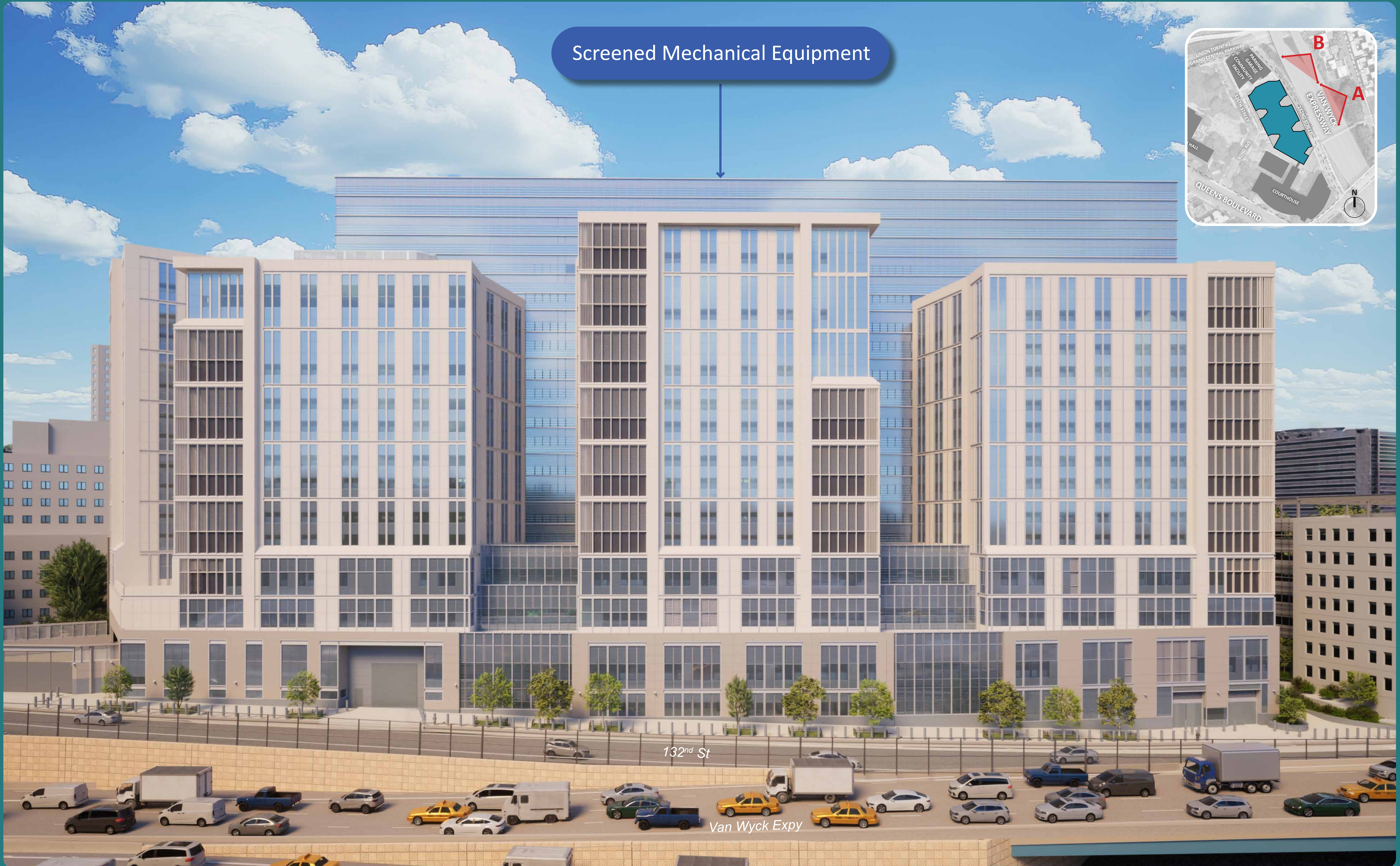
VIEW A - 132 ND STREET - EAST FACADE
