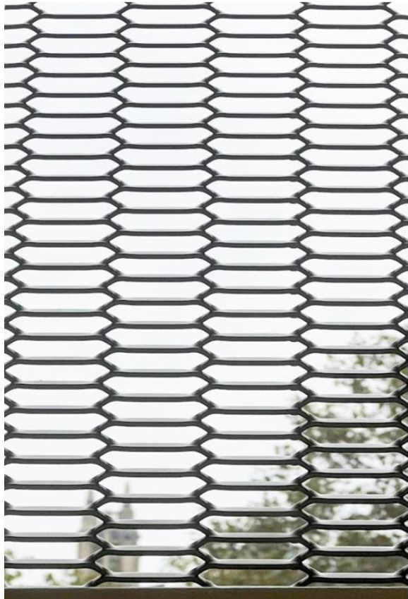
ARCHITECTURAL SCREEN LOOKING UP MAXIMIZING ACCESS TO OUTDOORS FOR PEOPLE IN CUSTODY
