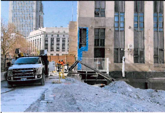
Photo 7: View of a sonic drill rig and a soil boring for the geotechnical investigation in progress.
