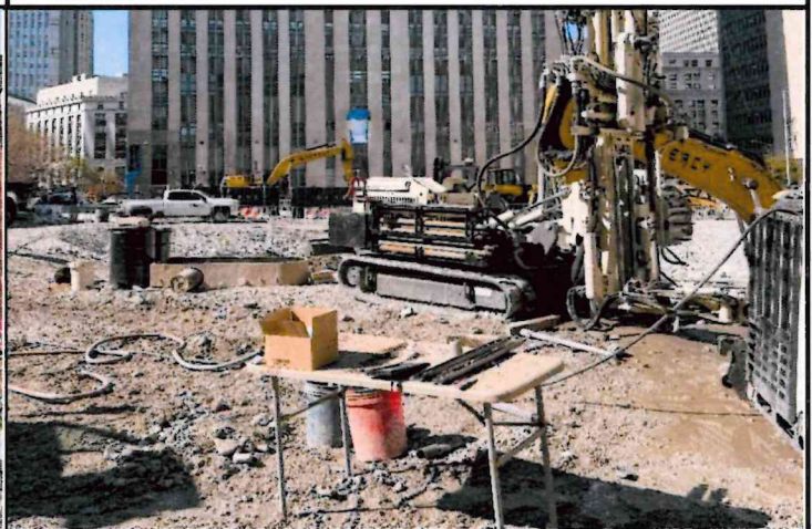
Photo 8: View of a Geoprobe drill rig and a soil boring and soil sampling for the geotechnical investigation in progress.
