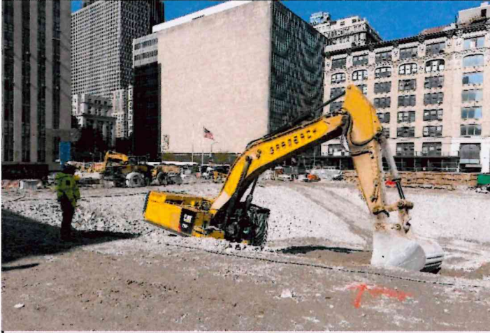
Photo 11: View of an excavator working on grading to facilitate access to drill rigs for the geotechnical investigation.
