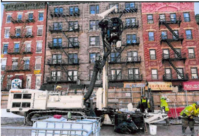
Photo 7: View of a sonic drill rig and a soil boring for the geotechnical investigation in progress.
