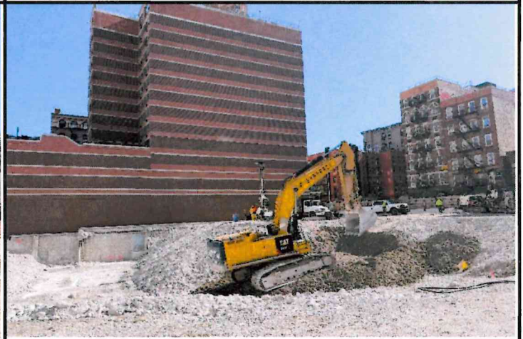
Photo 12: View of an excavator working on grading to facilitate access to drill rigs for the geotechnical investigation.
