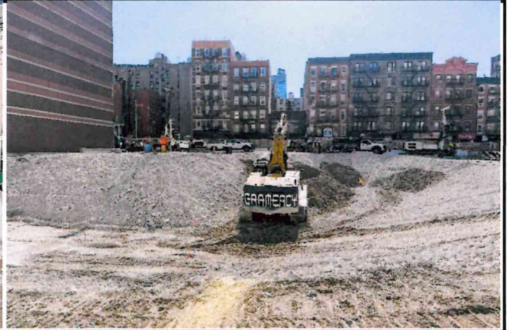
Photo 12: View of an excavator working on grading to facilitate access to drill rigs for the geotechnical investigation.
