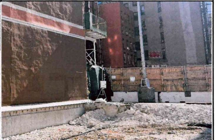
Photo 4: View of the northeast corner of the interior of the Site showing the onsite, downwind CAMP station set up for the geotechnical investigation.
