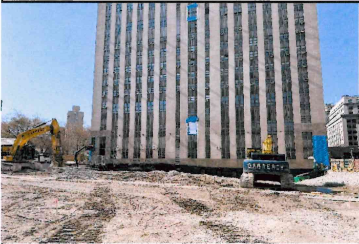
Photo 11: View of an excavator working on grading to facilitate access to drill rigs for the geotechnical investigation.
