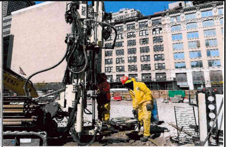
Photo 8: View of a Geoprobe drill rig and a soil boring and soil sampling for the geotechnical investigation in progress.
