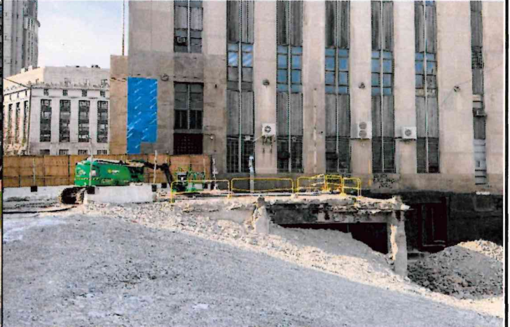
Photo 4: View of Chung Pak south wall showing North Tower Gym Wall removed and filled former basement area, 03-12-2025.
