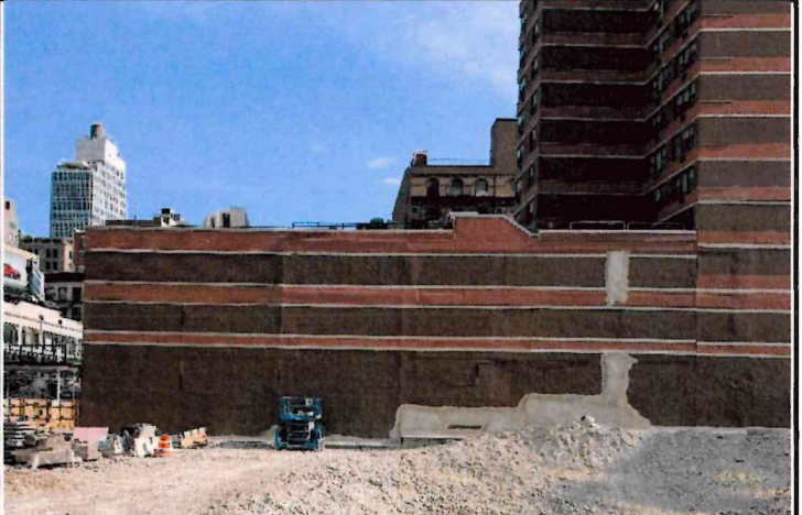
Photo 4: View of Chung Pak south wall showing North Tower Gym Wall removed and filled former basement area, 03-12-2025.
