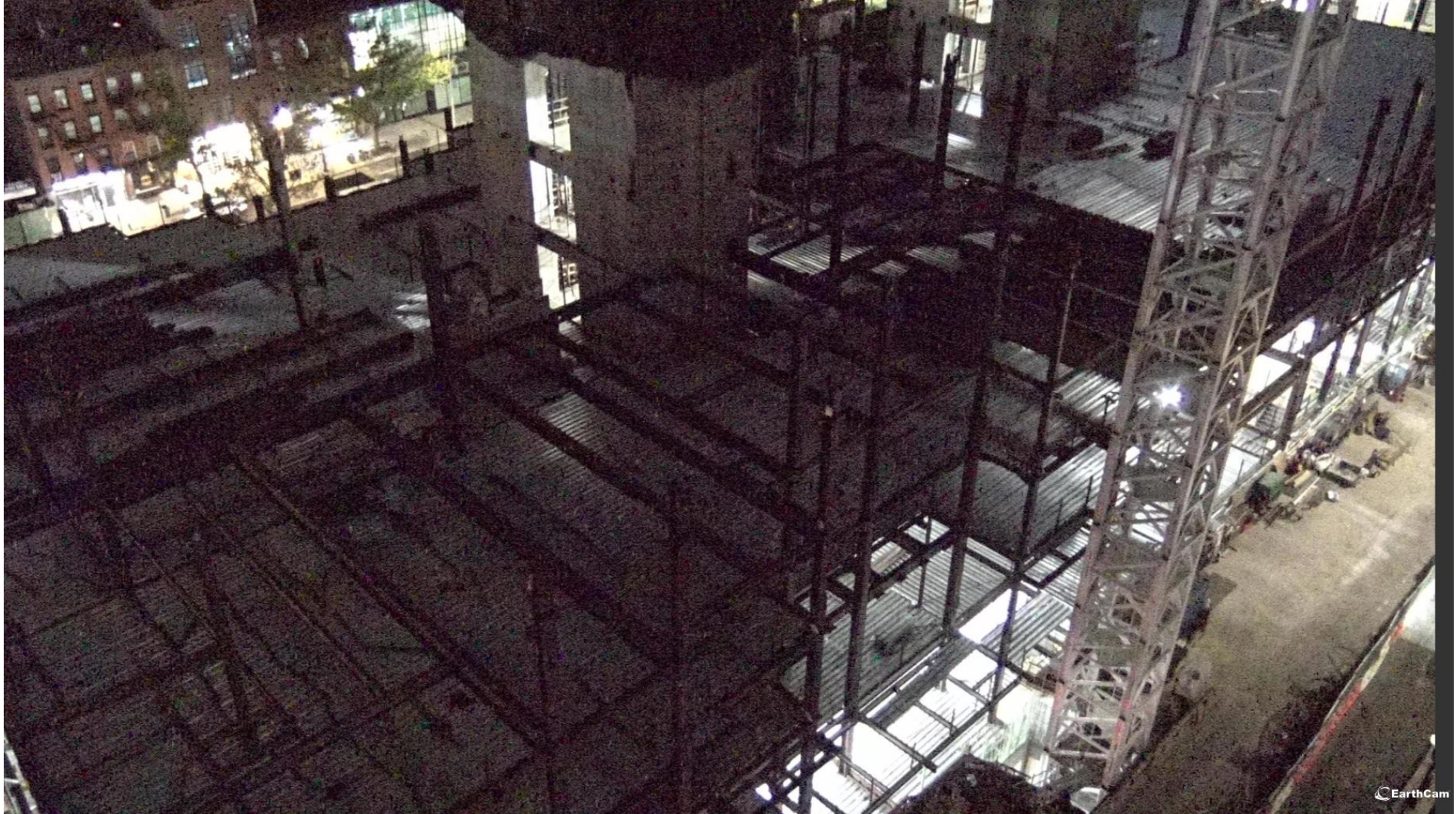
State Street looking Southwest
