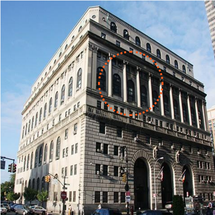
KINGS COUNTY CRIMINAL COURTHOUSE
