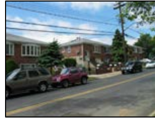
23rd Avenue between 128th and 129th streets - semi-detached two-family development R4-1 proposed
