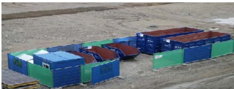
Photo of construction waste collection bins where waste can be separated
