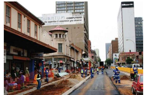
Construction on the Rea Vaya Project
