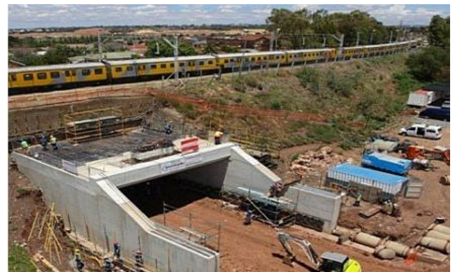
Work on Phase 2 Continues
