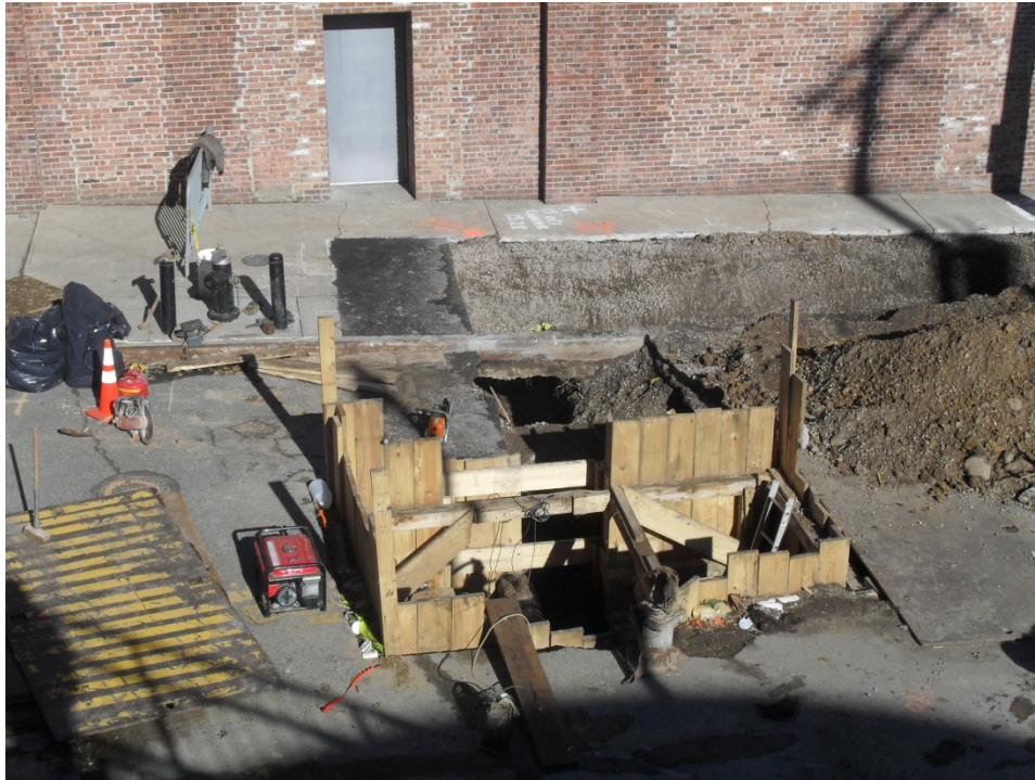
Relocation of gas line on Victory Boulevard, east of SIRR tracks
