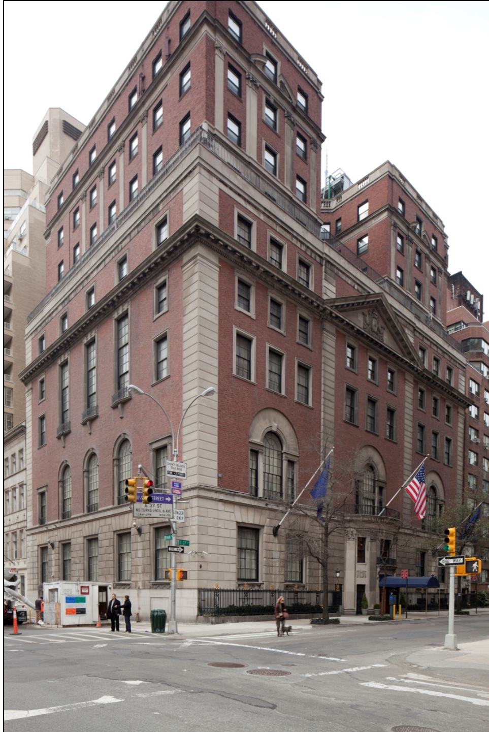
Union League Club 38 East 37 th Street (aka 34-38 East 37 th Street), 48 Park Avenue) Borough of Manhattan Tax Map Block 866, Lot 42 East/North façades, viewed from Park Avenue Photo by Christopher D. Brazee
