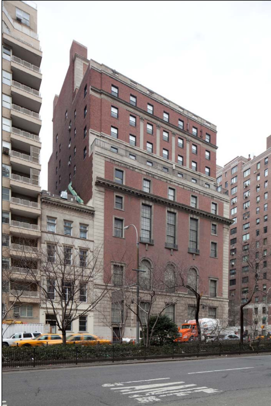
Union League Club South/East facades, view from Park Avenue Photo: Christopher D. Brazee, 2011
