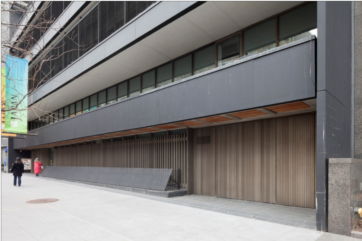
Japan Society Headquarters First story from west (top), from east (bottom) Photos: Christopher D. Brazee, 2011
