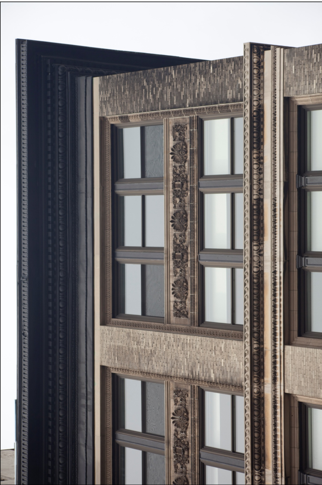
Rogers, Peet & Company Building Detail of terra-cotta spandrel and molded cornice Photo: Christopher D. Brazee, 2010
