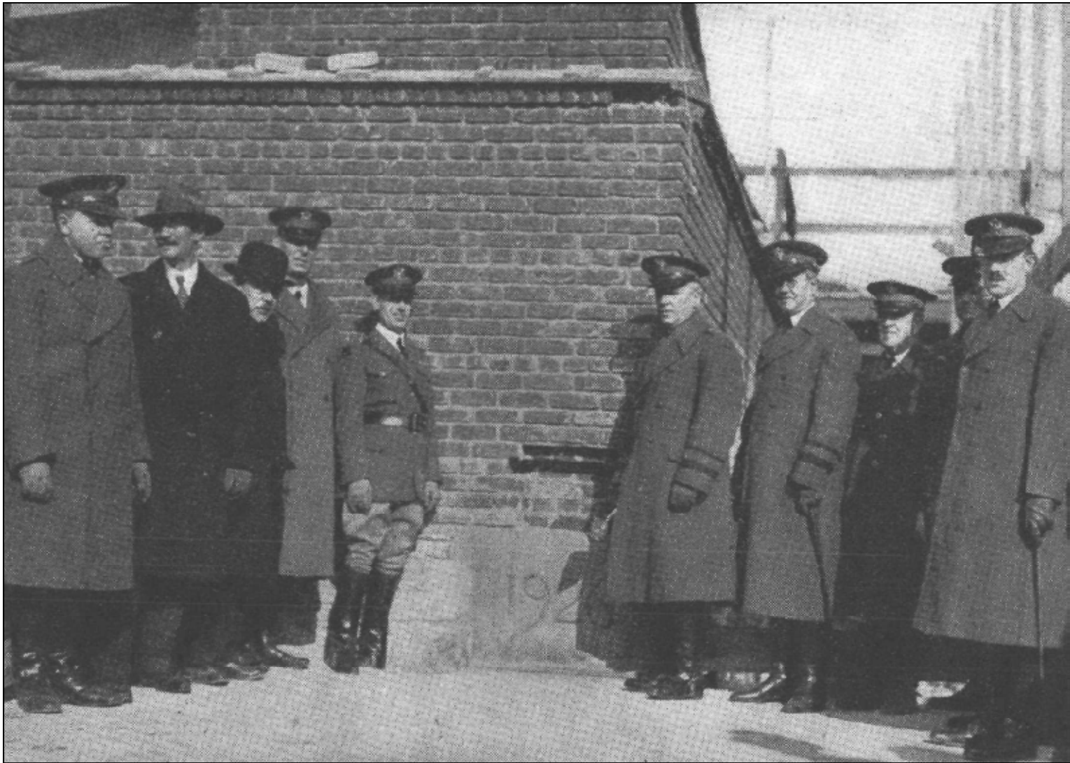
Cornerstone laying of the Headquarters Troop, 51st Cavalry Brigade Armory, March 5, 1927 Architect August Windolph is third from left Source: "General Haskell Lays Corner Stone," New York National Guardsman (April 1927), 7.
