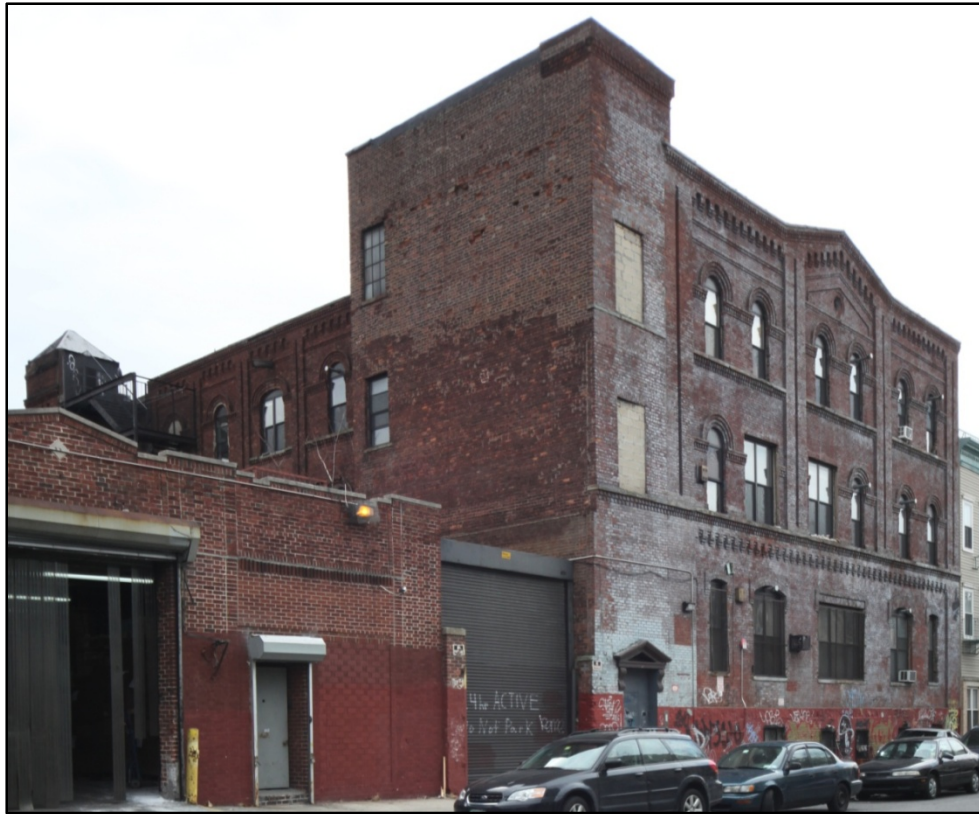
William Ulmer Brewery Stable and Storage Building, Northeast and Northwest Facades Photo: Christopher D, Brazee, 2009
