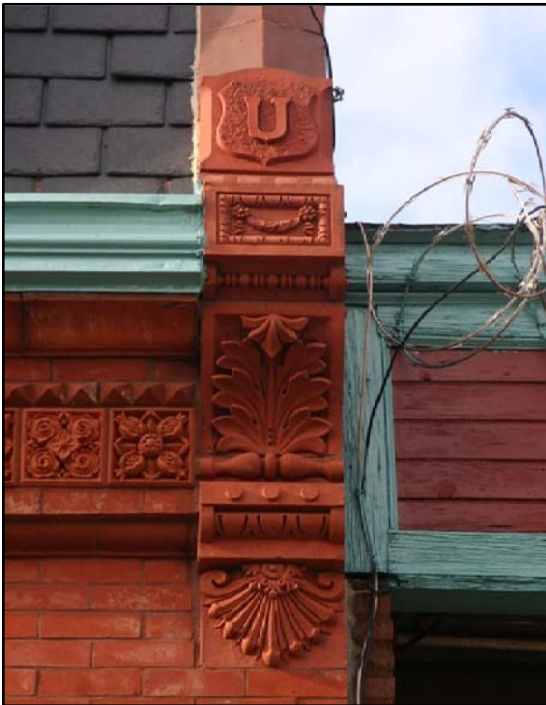
William Ulmer Brewery Office Building, Terra-Cotta Details Photos: Tara Harrison, 2009
